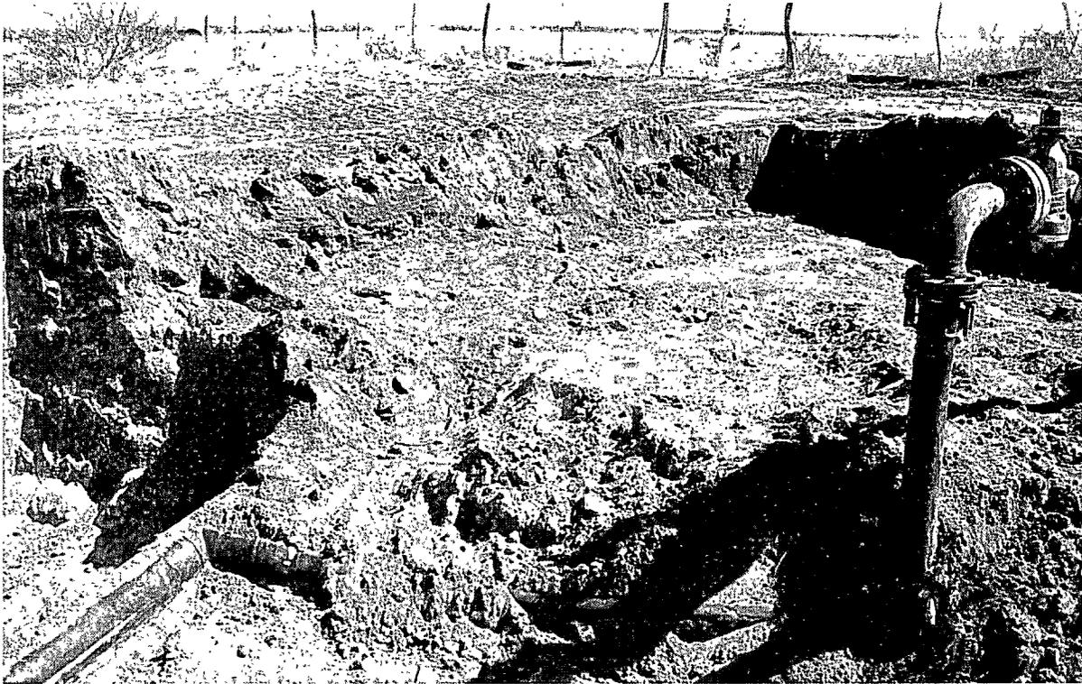
Site Photograph of Excavation and exposed 8 " Pipeline at the MA-4 8" release site.
