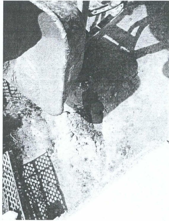
Plugging the well with bentonite/concrete slurry
