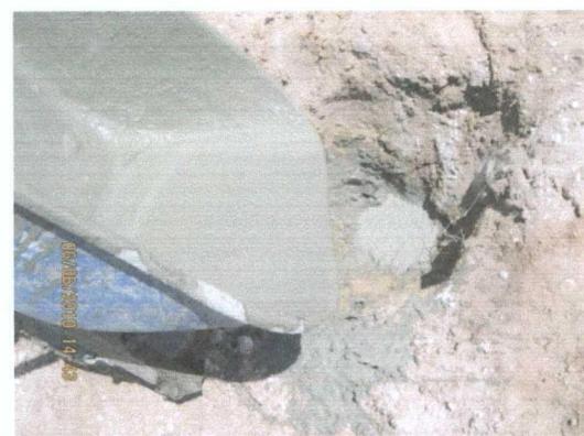
plugging RW-1 with bentonite/cement slurry
