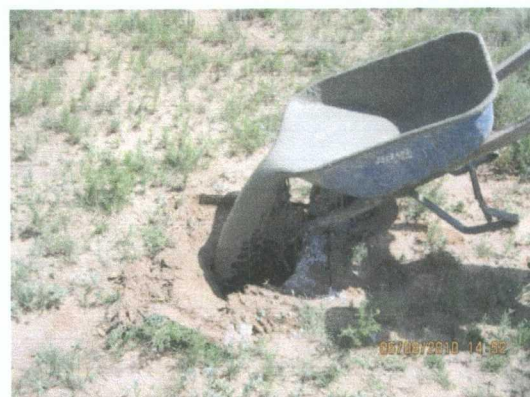
plugging MW-4 with bentonite/cement slurry
