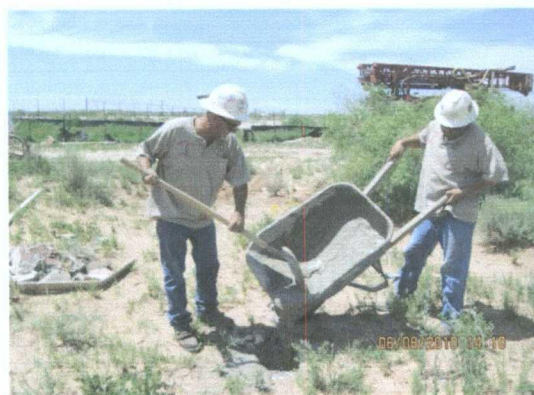
plugging MW-2 with bentonite/cement slurry
