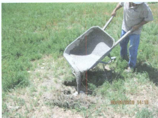
plugging MW-1 with bentonite/cement slurry
