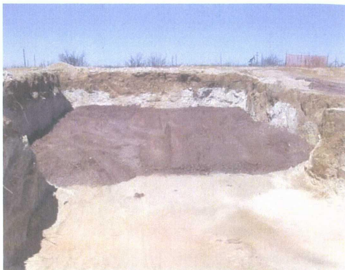
Second clay layer (40 ft by 50 ft) at 12 ft bgs (04-07-09)
