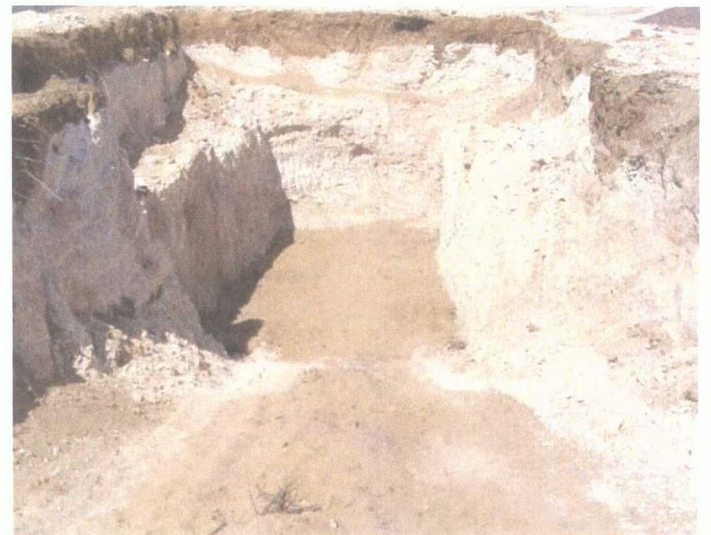
Sand layer above first plastic layer (04-06-09)
