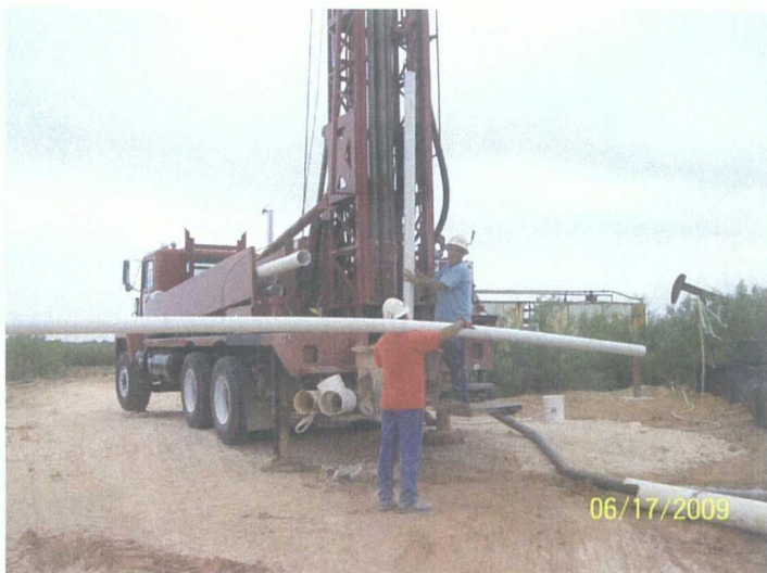
Placing the casing
