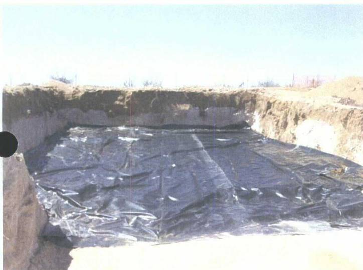
Plastic liner above second clay layer at 11 ft bgs (04-07-09)
