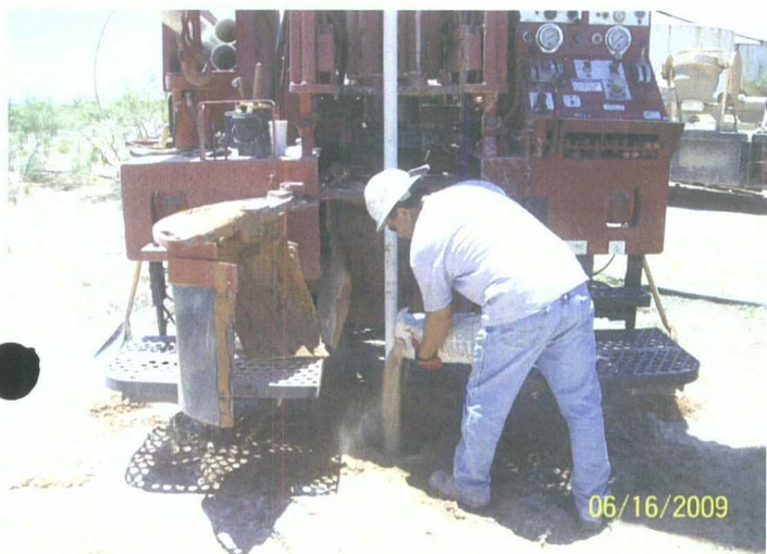
Putting in the sand filter
