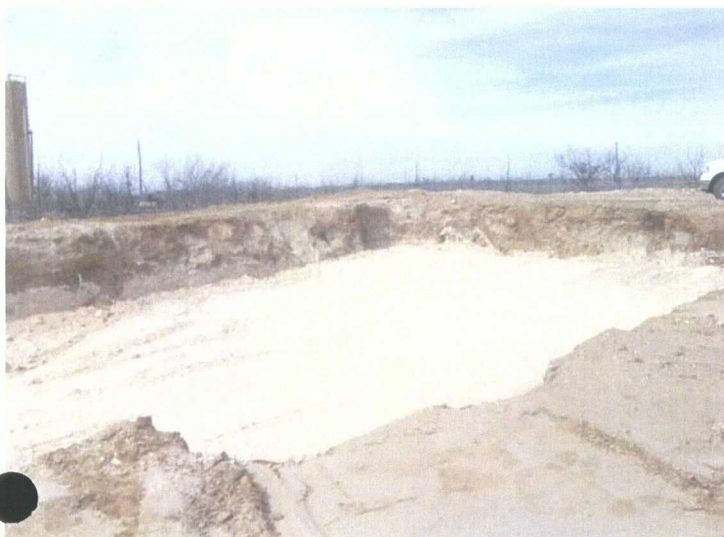
Caliche backfill up to ~5 ft bgs (04-08-09)
