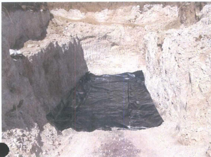
Plastic liner above first clay layer at 29 ft bgs (04-06-09)
