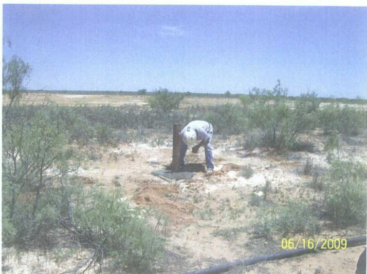
Concreting the well in
