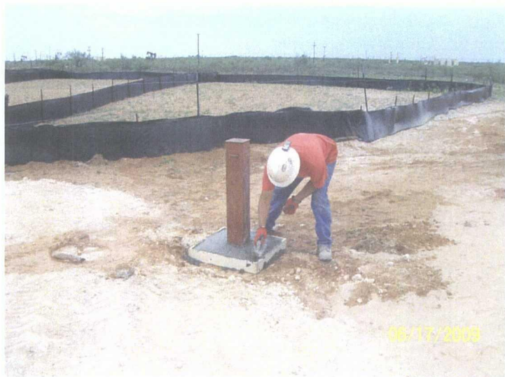
Concreting the well in
