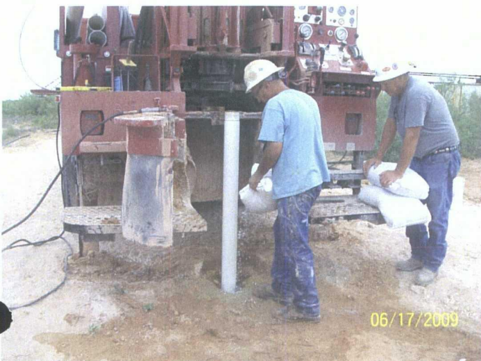
Sealing the well with bentonite
