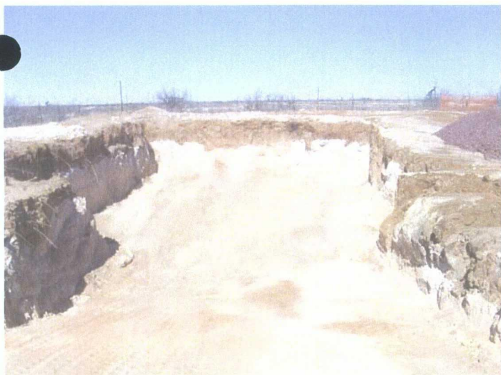
Caliche backfill up to ~12 ft bgs (04-07-09)
