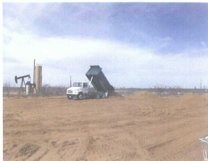
Sand layer up to surface grade (04-14-09)
