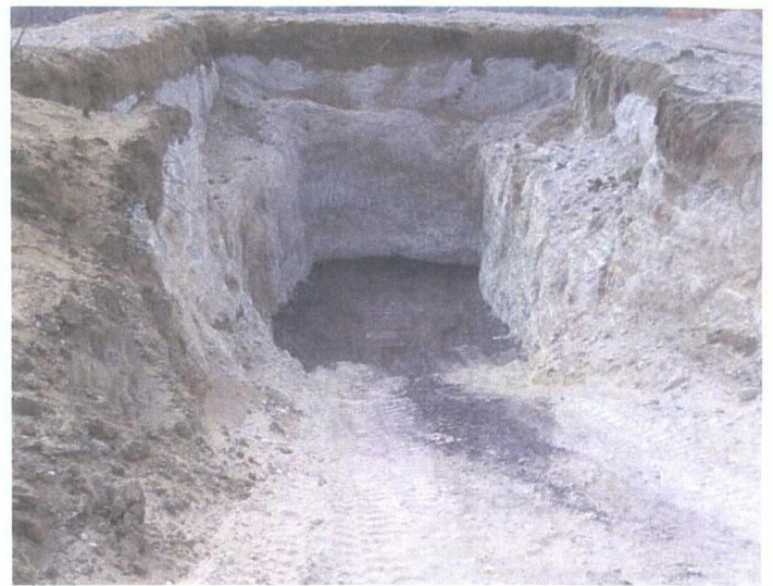
First clay layer (20 ft by 40 ft) at 30 ft bgs (04-01-09)
