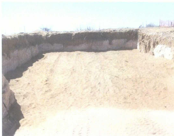
Sand layer above second plastic layer (04-07-09)
