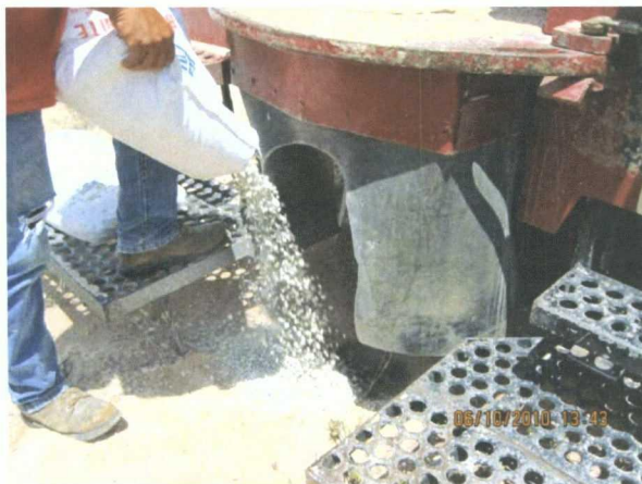
plugging SB-9 in total with bentonite
