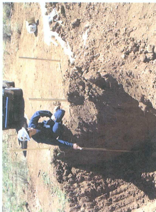
Photo 35. B8 new - Excavated to 5' bgs, shovel in picture is 4' 9", 51/52 stakes in place
