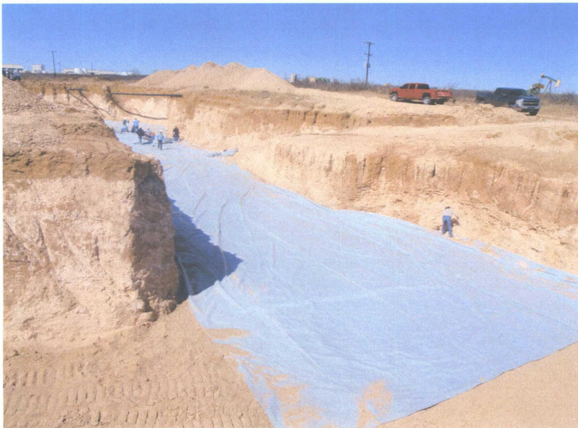
SUG Red Byrd 8-Inch Monument Release Site, During Polyliner Installation
