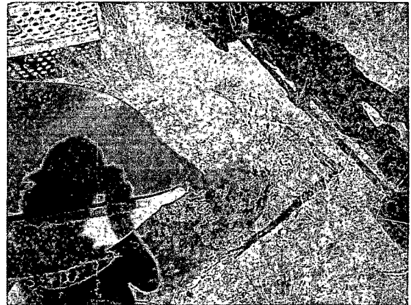
Plugging the well with 1-3% bentonite/concrete slurry
