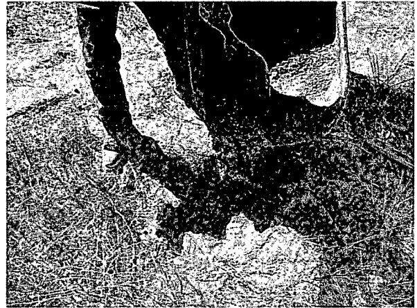
Plugging the well with 1-3% bentonite/concrete slurry
