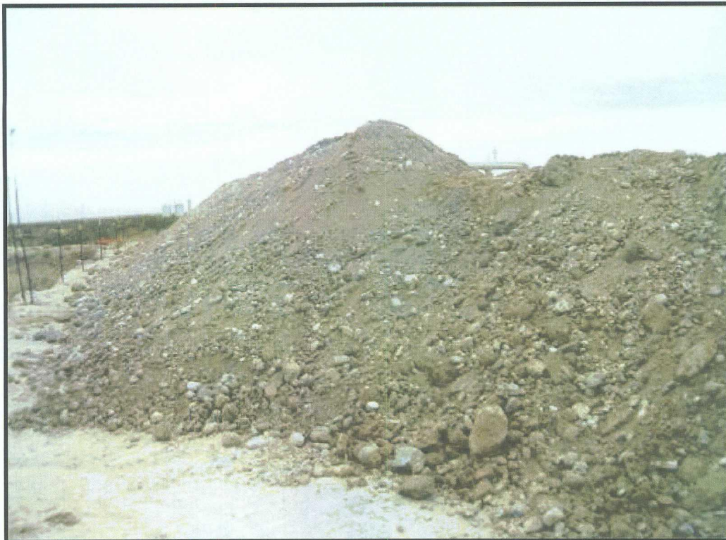
Highly stained soils stockpiled facing west
