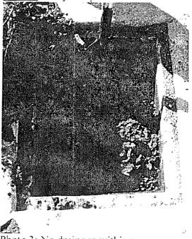
Photo 3: No drainage within sump.
