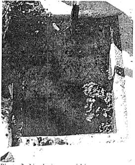
Photo 3: No drainage within sump.
