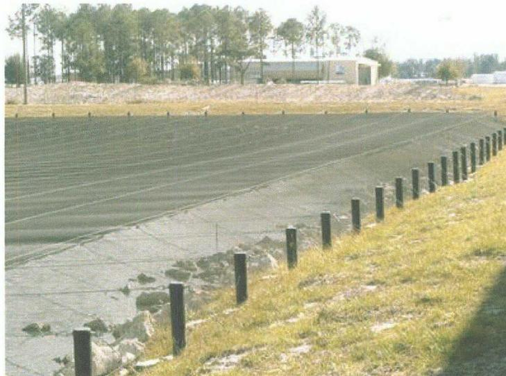
This system has proven to withstand snow and wind loads while effectively hiding the water surface from the view of migratory birds.
