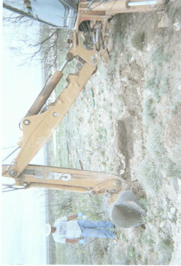
Delineation trench being excavated
