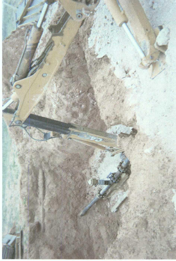
Delineation trench being excavated
