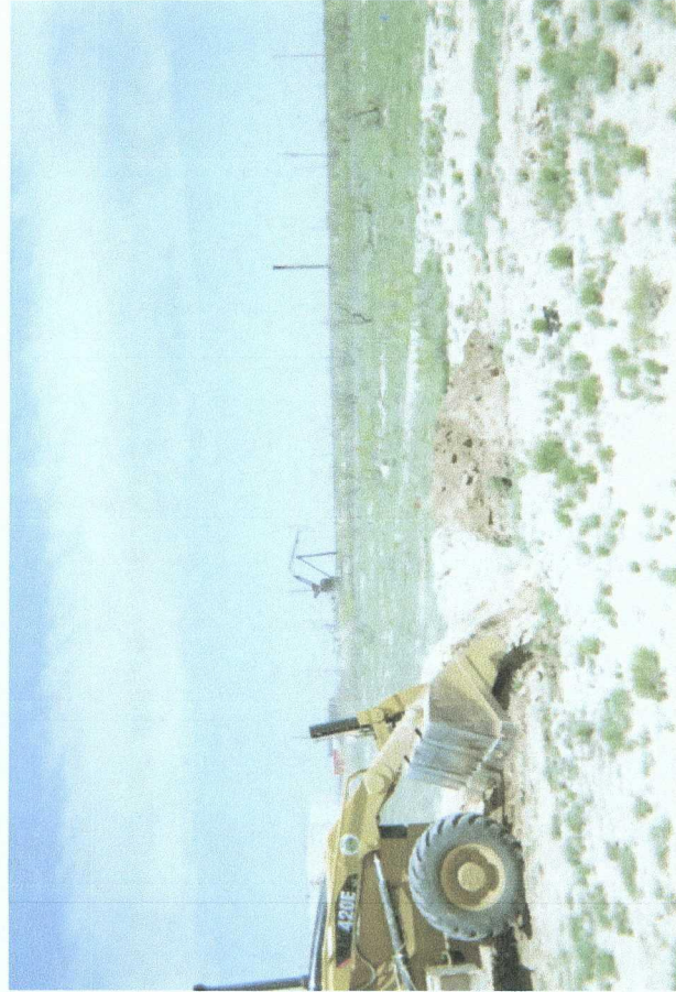
Backfilling excavation
