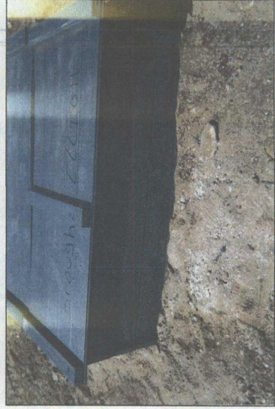
New Watertight Junction Box 45 ft Southeast
