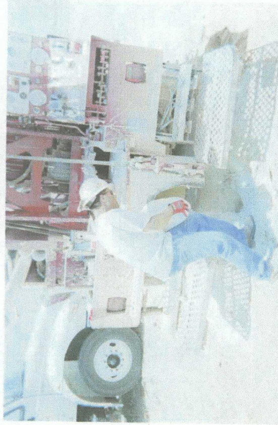
plugging SB #1 with bentonite
