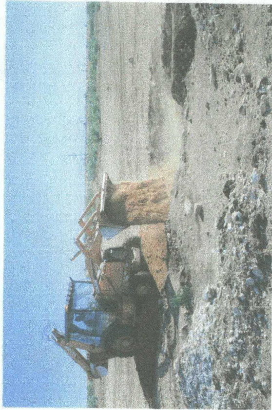
backfilling the former junction box prior to drilling
