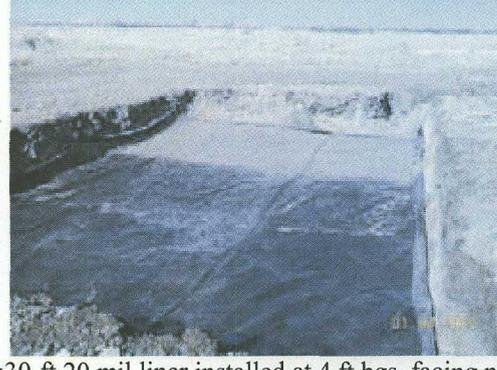
48x30-ft 20 mil liner installed at 4 ft bgs, facing north
