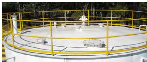
Figure 2.14: Fixed roof tank openings.
