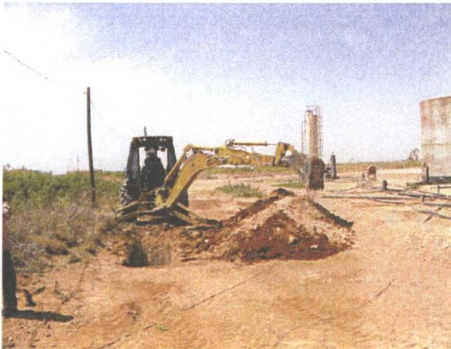
On May 6, 2001 a different backhoe was used to complete the excavations. The four deep trenches (D, E, F, and G) were excavated to depths of 12 to 15 feet, depending on the hardness of the soil encountered, in order to verify historic sampling results and establish a chloride concentration profile. All sampling of trenches was completed.
