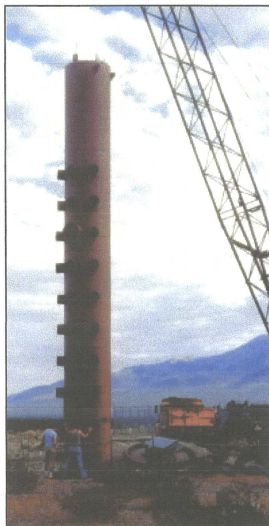
Figure 4. Installation of vertical shaft used for soil-moisture monitoring in upper 45 feet of unsaturated zone beneath undisturbed, vegetated area. Photograph by David S. Morgan, U.S. Geological Survey, August 1983.
