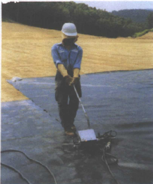
Joining the Seam of a Synthetic Liner
