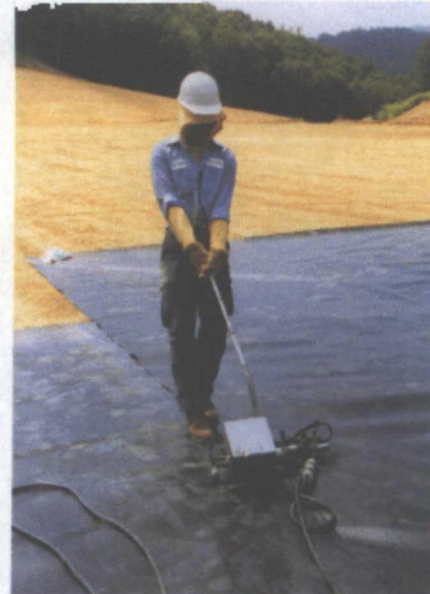
Joining the Seam of a Synthetic Liner
