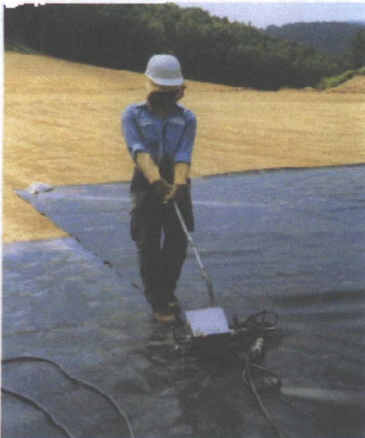
Joining the Seam of a Synthetic Liner
