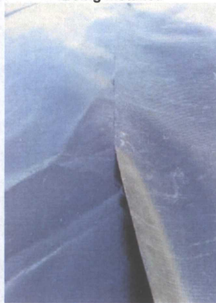
Example of a Synthetic Liner Being Installed
