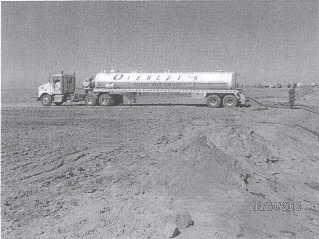
Well 47-07 (A-758-POD6) BLM Lease: vacuum tank emptying reservoir.
