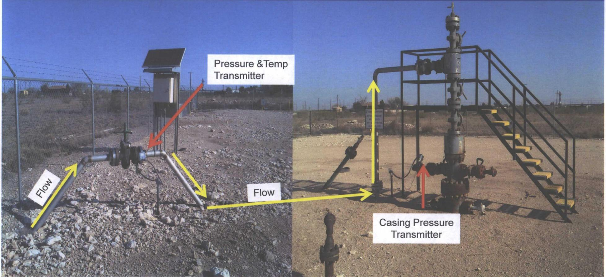
Pressure Transmitters are connected to the casing valve on all injection wells in NHU
