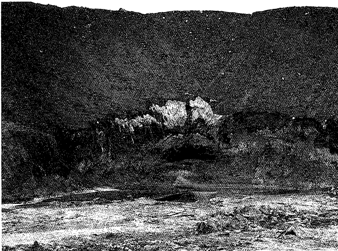
FIGURE I-25. CAVITATION BURN PIT.
