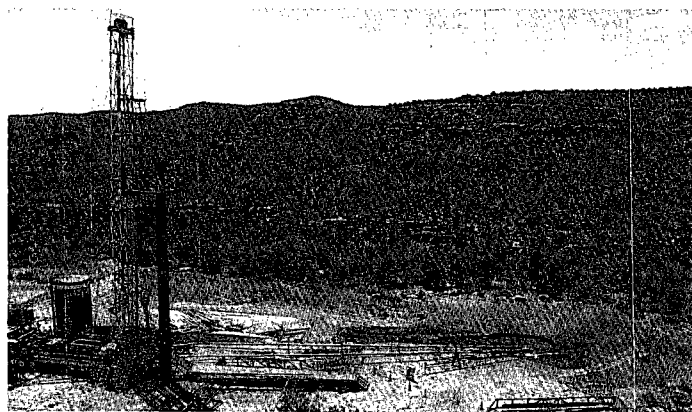
FIGURE I-39. TYPICAL COMPLETION WITH A FLARE BERM AND WASTE PITS. Photo by Dan Randolph
