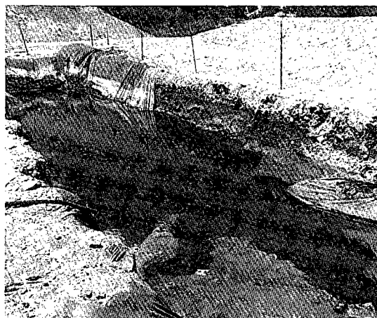
FIGURE I-21. TORN LINER ON AN OPEN PIT.
