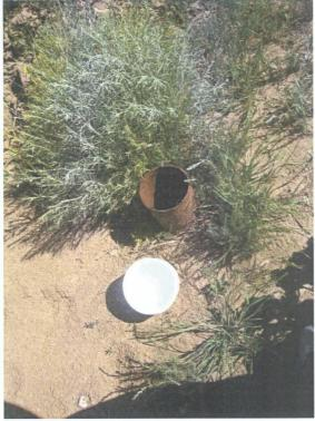
2. (Top of drill pad is approximately 4 feet above top of this well casing)
