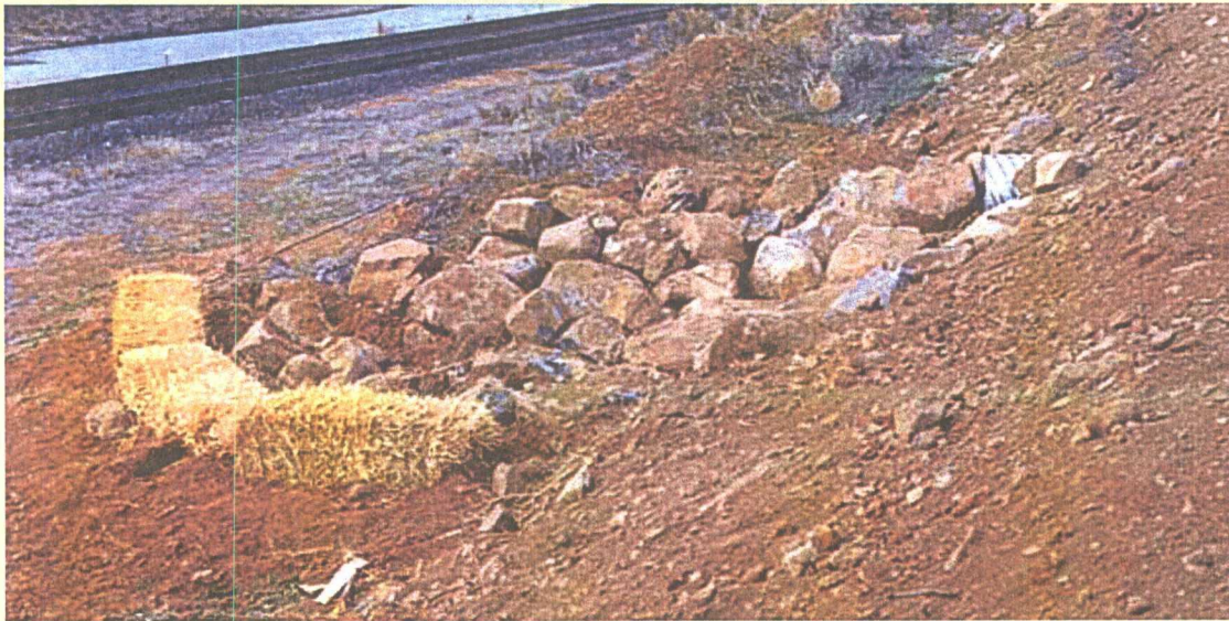
Properly sized rock rip-rap at culvert outlets helps reduce water velocity and resulting soil erosion.
