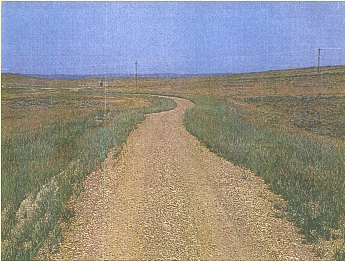
This example of interim road reclamation shows that reapplying topsoil and the regrowth of vegetation along the road borrow ditches of this resource road reduces the loss of forage, habitat, and sediment, decreases maintenance costs, and helps maintain the scenic quality.
