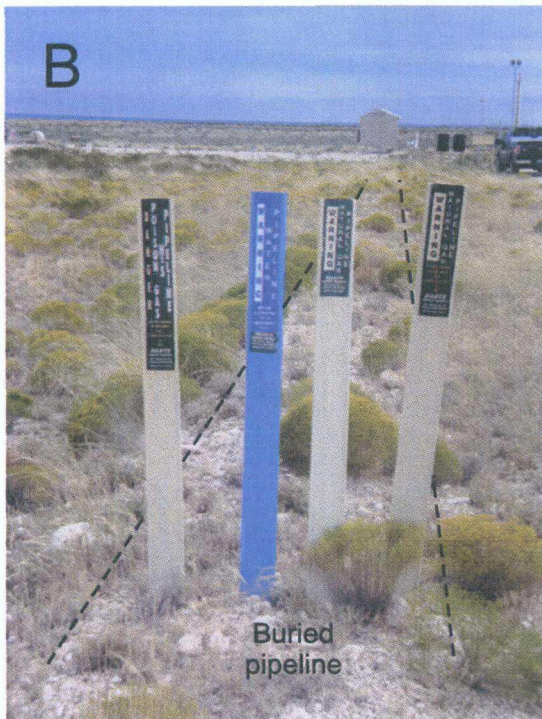
Figure 1: Photos of Pipeline Connecting Agave Energy's Dagger Draw Gas Plant With Metropolis Disposal #1 well. A) Acid Gas Compressed at the Gas Plant is Introduced to a 2" Stainless Steel Pipeline Surrounded by a 6" Polyethylene Pipe. Pipeline Integrity is Monitored Using a Stream of Sweet Natural Gas in the Volume Between the Two Pipes. B) Outside of the Fenced in Areas at the Plant and Wellhead, the Pipeline is Buried and Clearly Marked. C) The Pipeline Rises Above Ground and Connects to the Production Tree at the Metropolis Disposal #1 Wellhead
