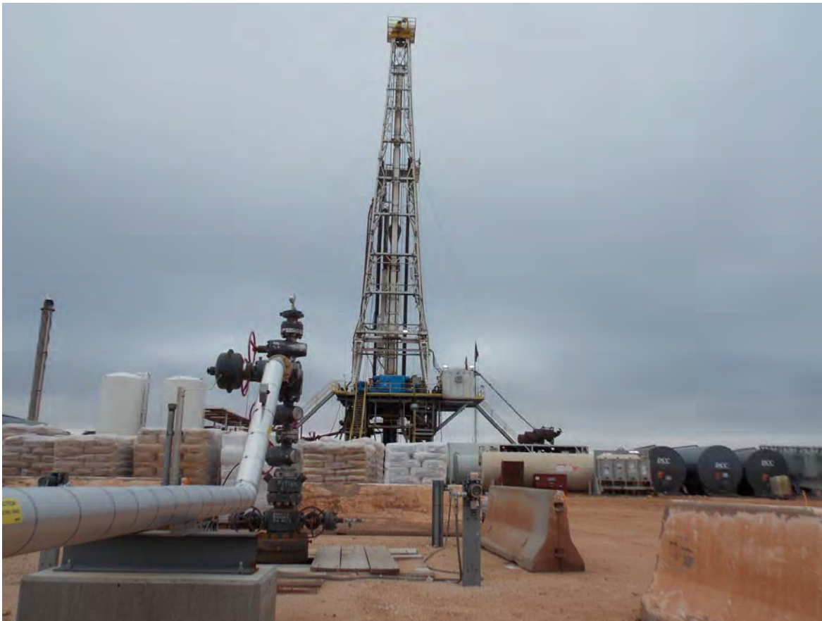
Figure 1 – Preparing to drill 12 ¼-inch borehole. Zia AGI #1 is in the foreground.
