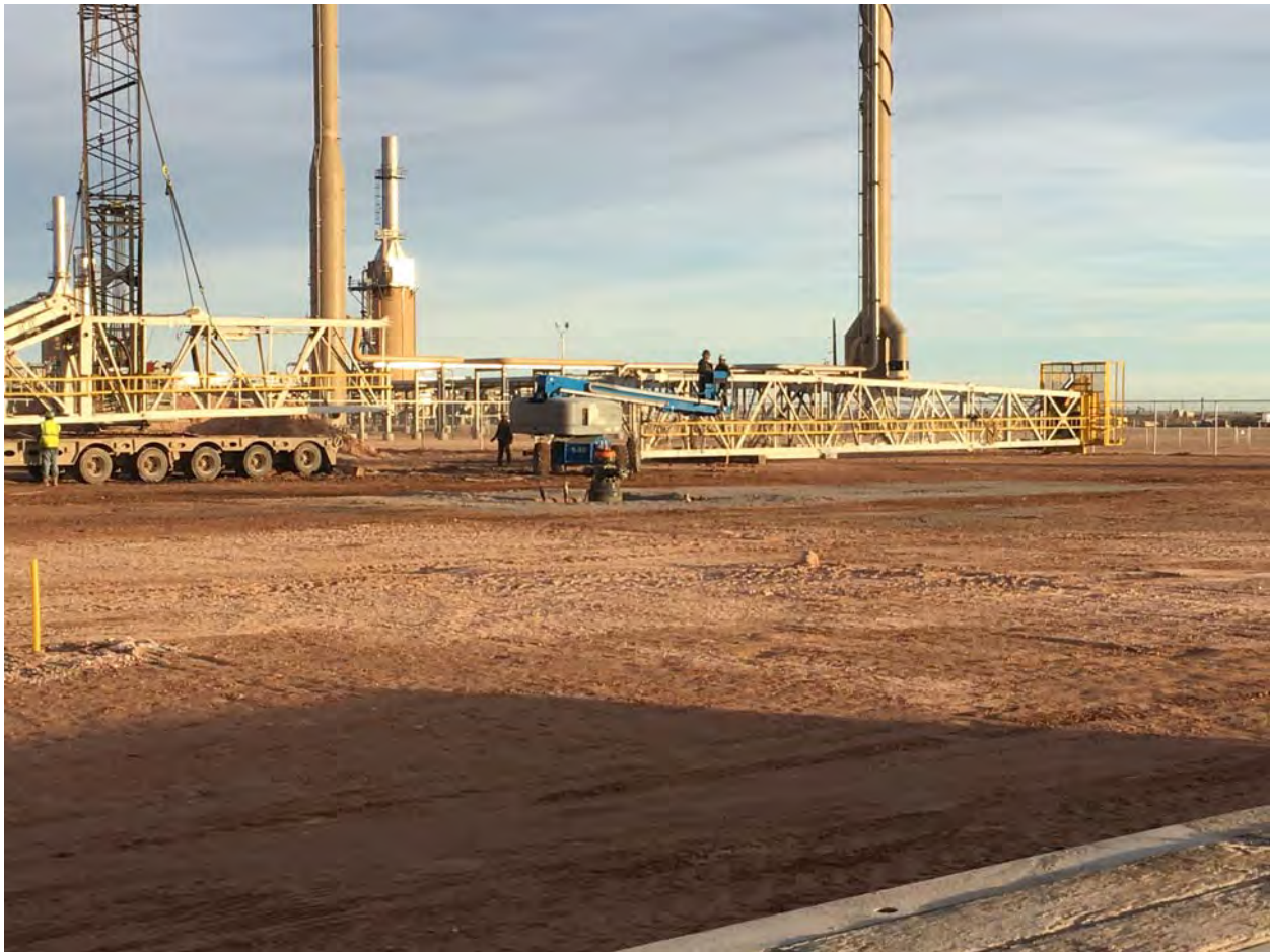
Figure 1: Demobilization of the Scandrill Freedom Rig. Zia AGI D #2 is in the foreground.
