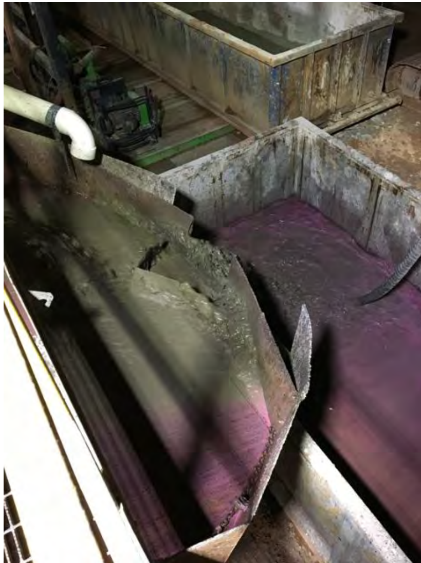
Figure 1A – Circulation of First Stage Cement of the 2 nd intermediate casing (144 sacks to surface). Photograph taken immediately after cement was first observed at the surface.
