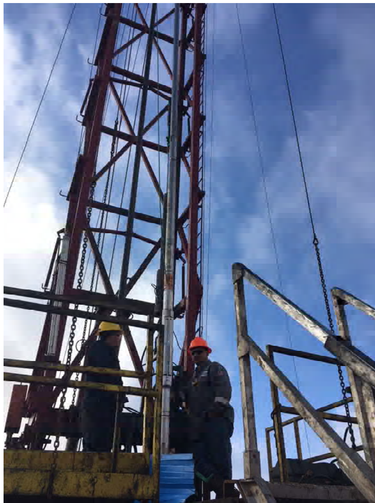
Figure 1: P/T gauge being installed.
