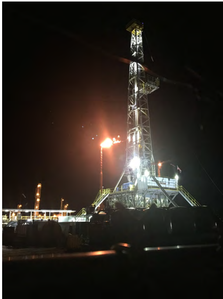
Figure 1 – Drilling the 12 ¼-inch 2 nd intermediate casing borehole. Plant flare is in the background.
