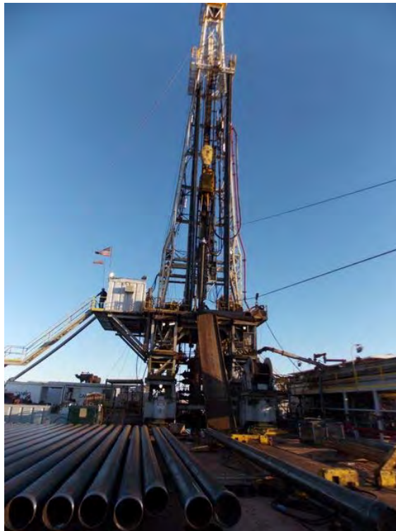
Figure 1 – Installing 1 st intermediate casing
