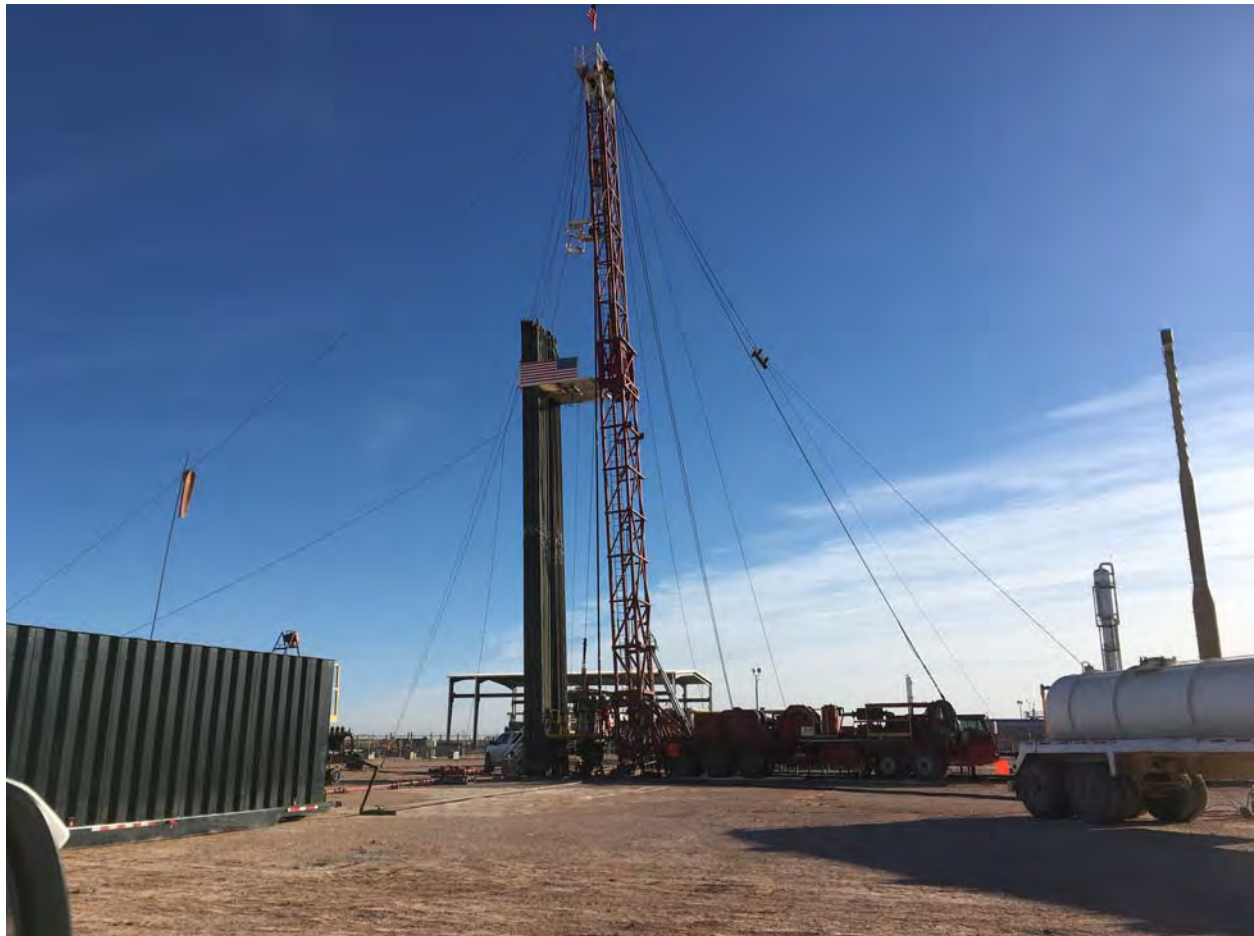
Figure 1: Standing Pipe at Workover Rig. Ready to TIH with Packer.
