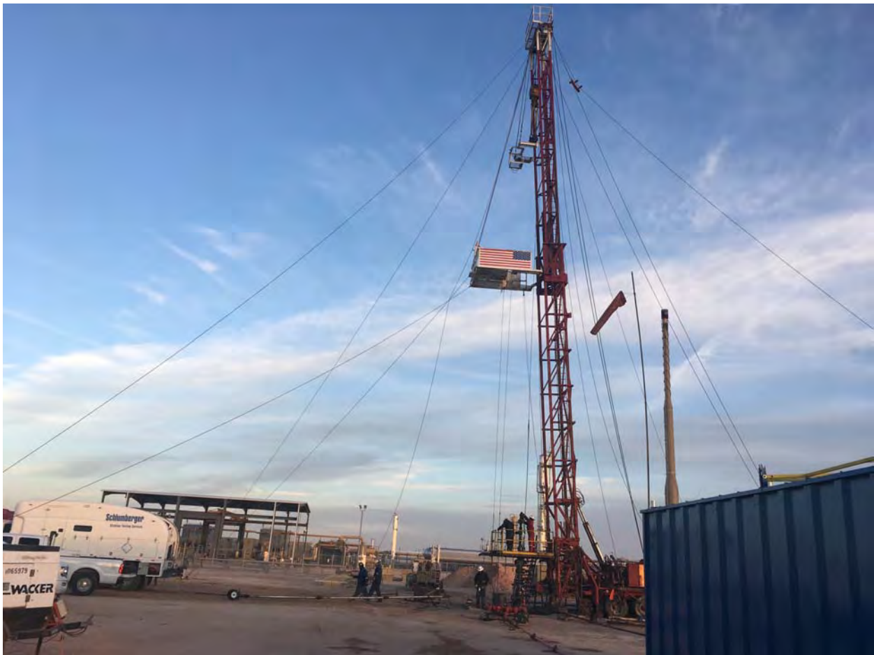
Figure 1: Schlumberger running P-T slickline.
