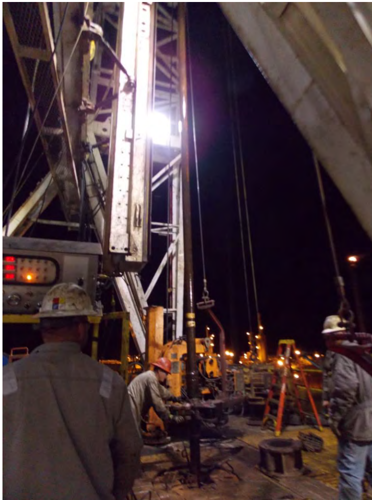
Figure 1 – Making Connections for the 17 ½-inch borehole
