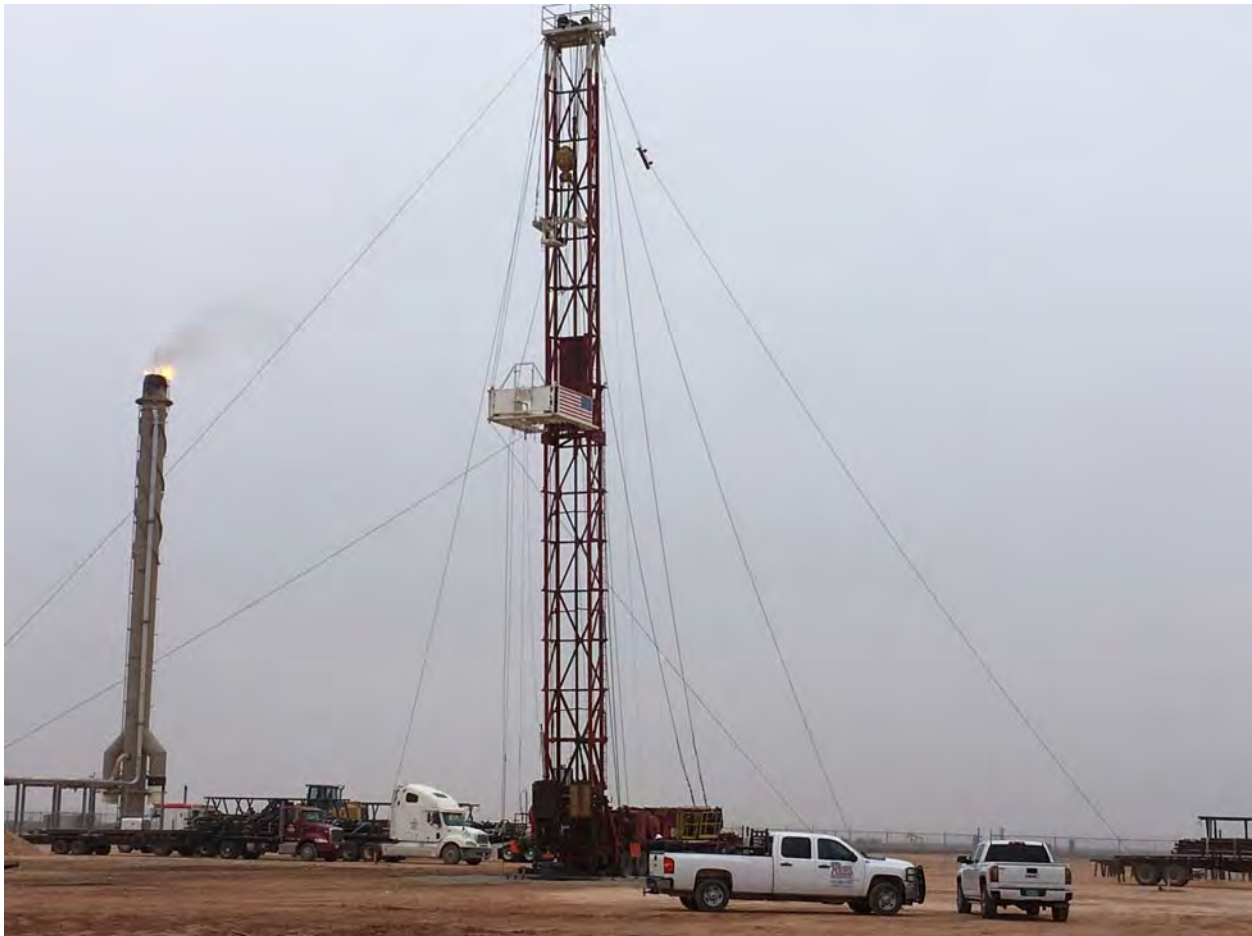
Figure 1: Workover rig in place and ready to begin completion procedures.
