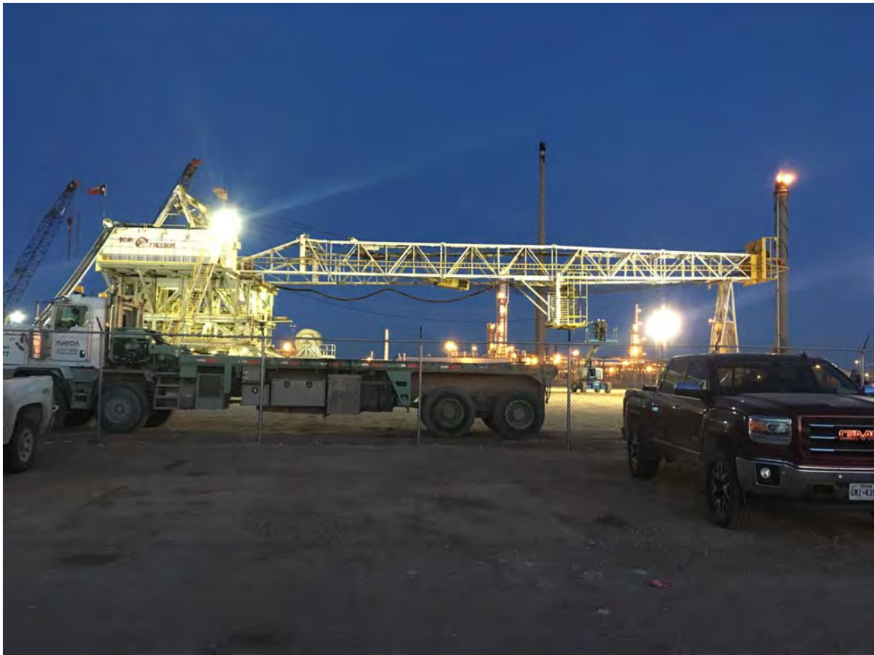
Figure 1: Demobilization of the Scandrill Freedom Rig.
