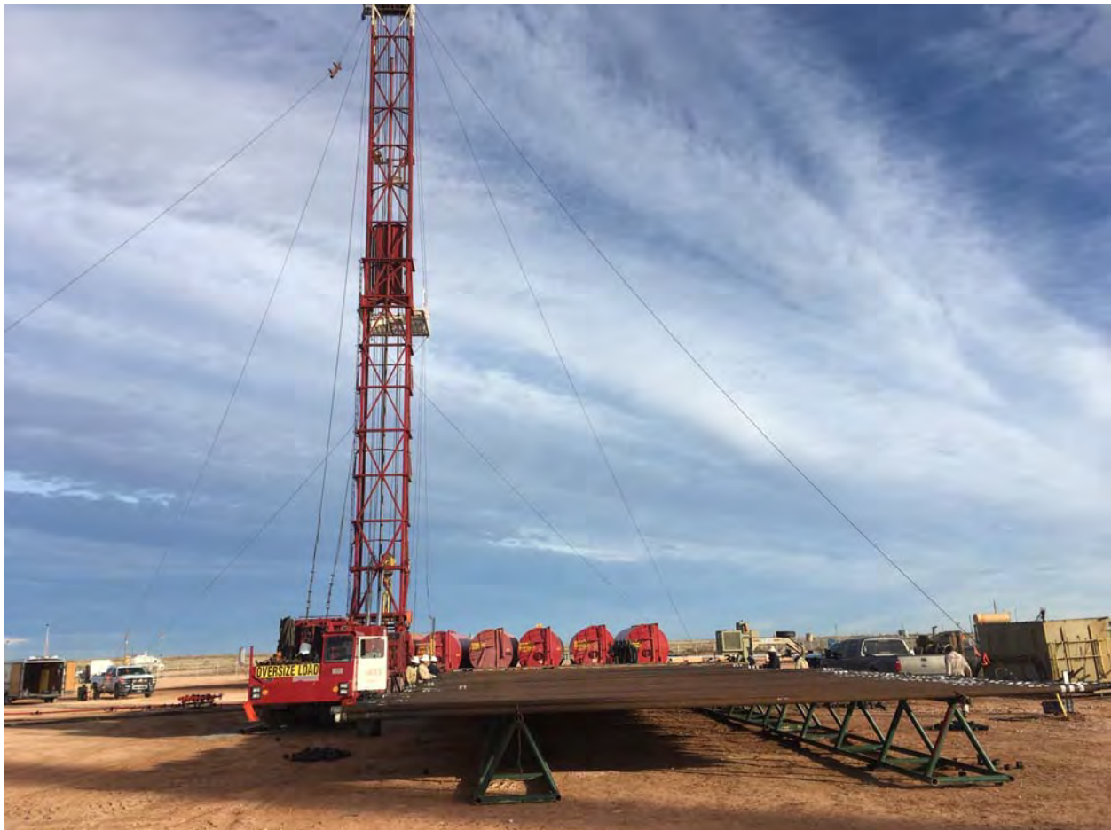
Figure 1: Preparing to trip in hole to drill out composite plug.
