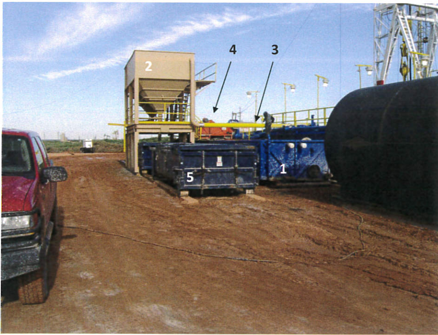
Closed Loop Drilling System: Mud tanks to right (1) Hopper in air to settle out solids (2) Water return pipe (3) Shaker between hopper and mud tanks (4) Roll offs on skids (5)
