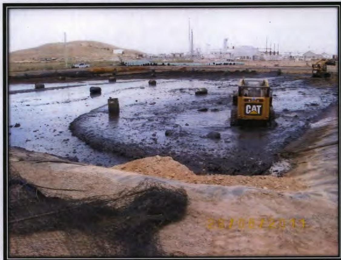
Photo 4 - Evaporation Pond during Solidification Process
