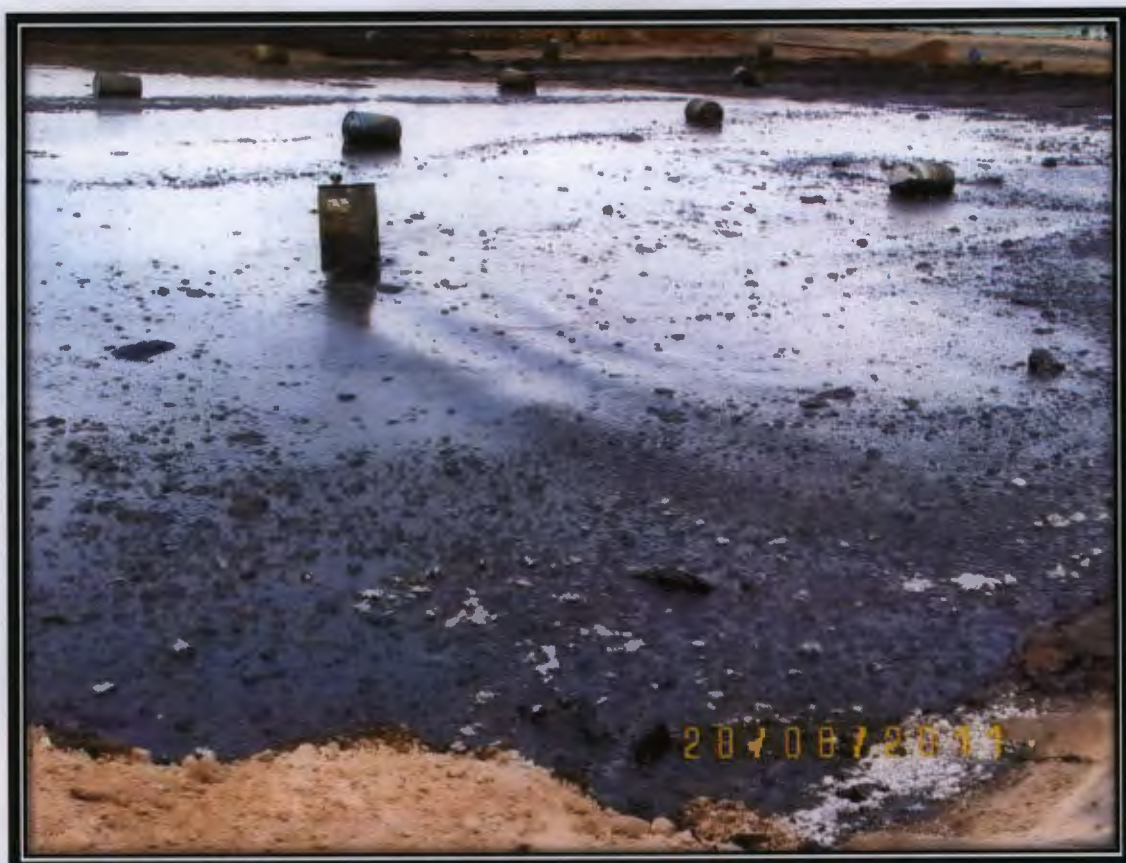
Photo 3 - Evaporation Pond at the Start of Solidification Process
