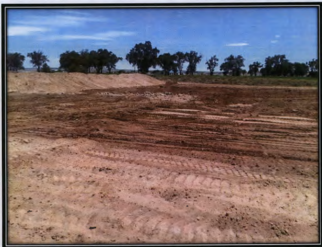
Photo 23 - Backfilling of Former Pit
