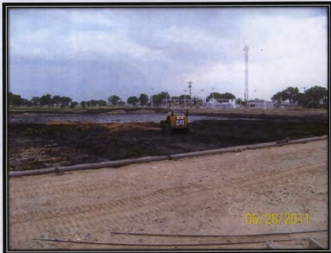
Photo 8 - Solidification of Evaporation Pond
