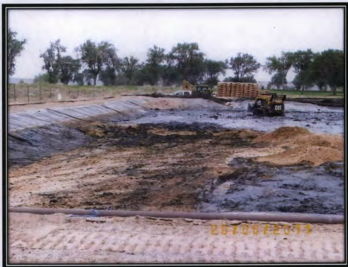
Photo 5 - Evaporation Pond during Solidification
