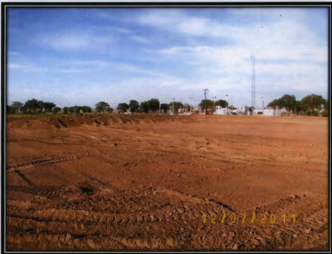
Photo 18 - Pit Bottom after Removal of Liner
