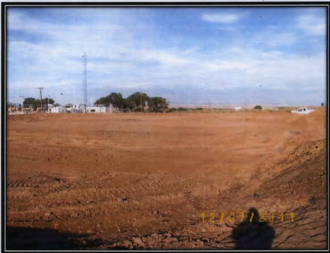
Photo 17 - Pit Bottom after Removal of Liner
