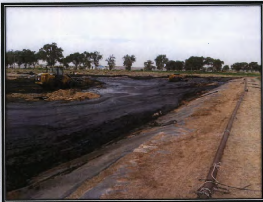
Photo 9 - Solidification of Evaporation Pond
