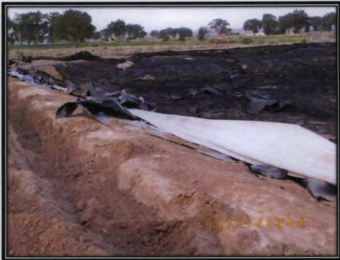
Photo 13 - Removal of Pit Liner Edge along East Side
