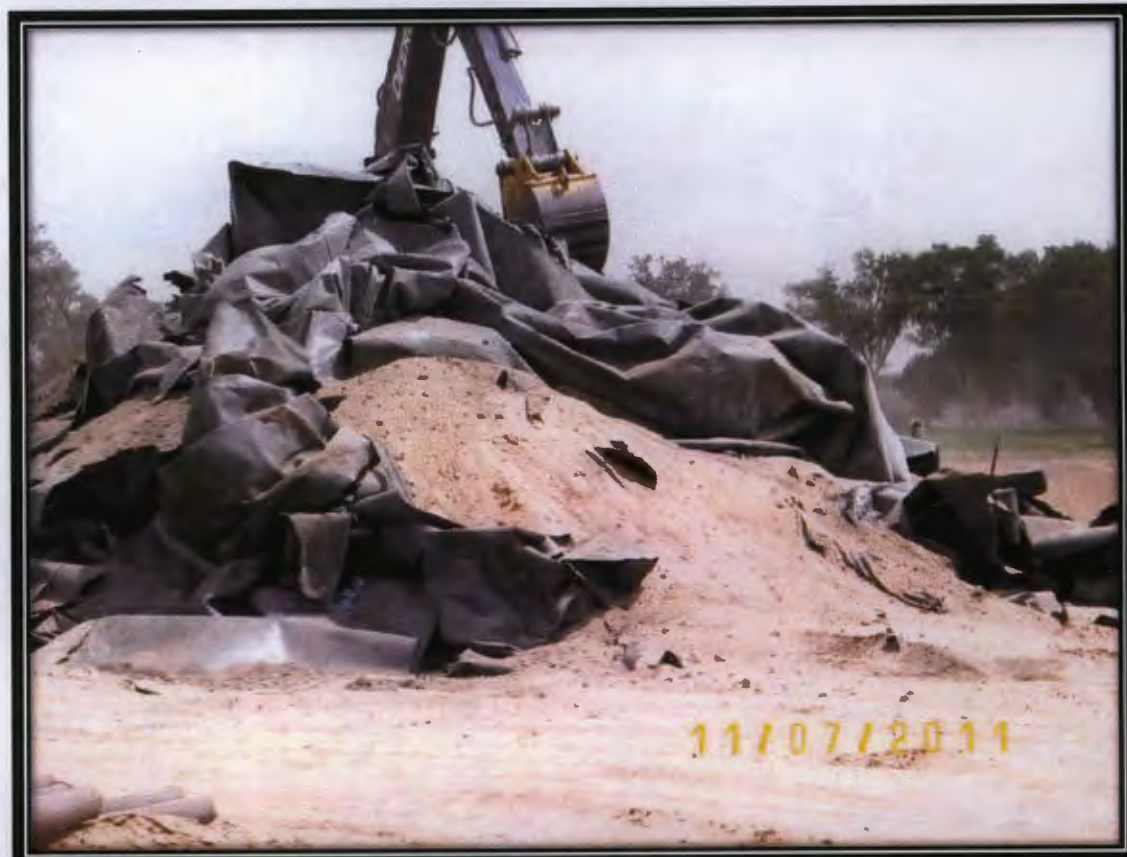
Photo 16 - Stockpiled Liner and Contaminated Soil
