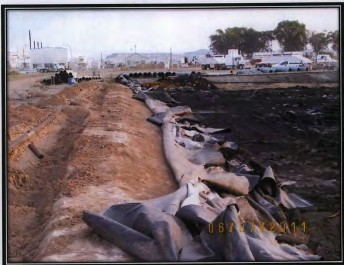
Photo 15 - Removal of Pit Liner Edge along West Side
