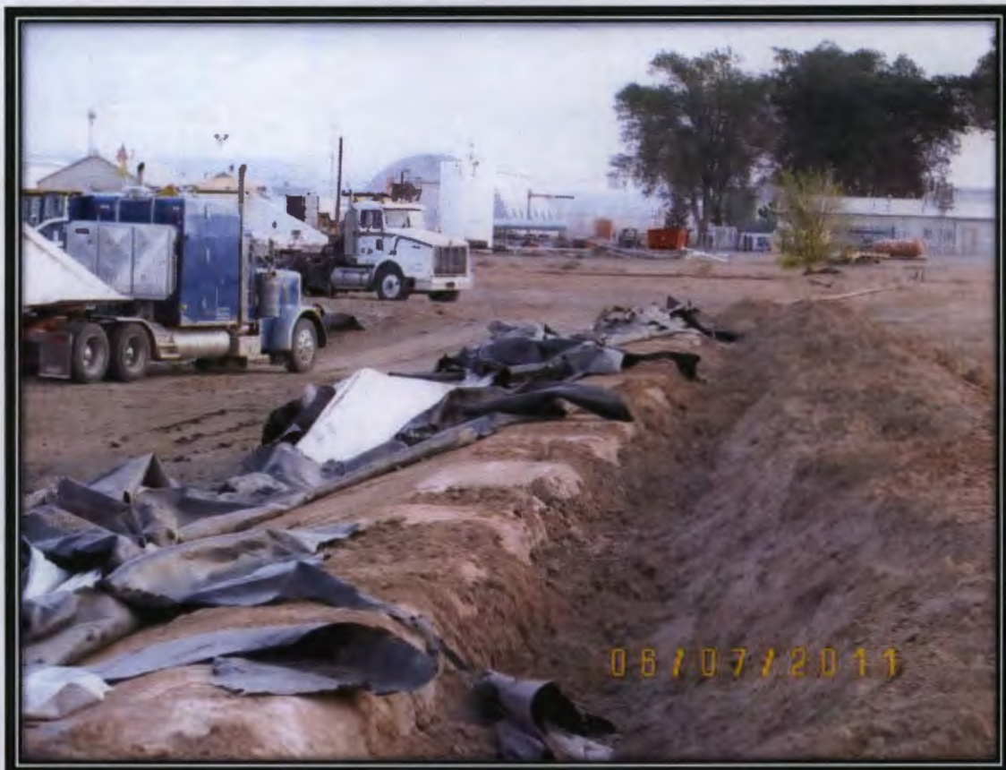
Photo 14 - Removal of Pit Liner Edge along West Side
