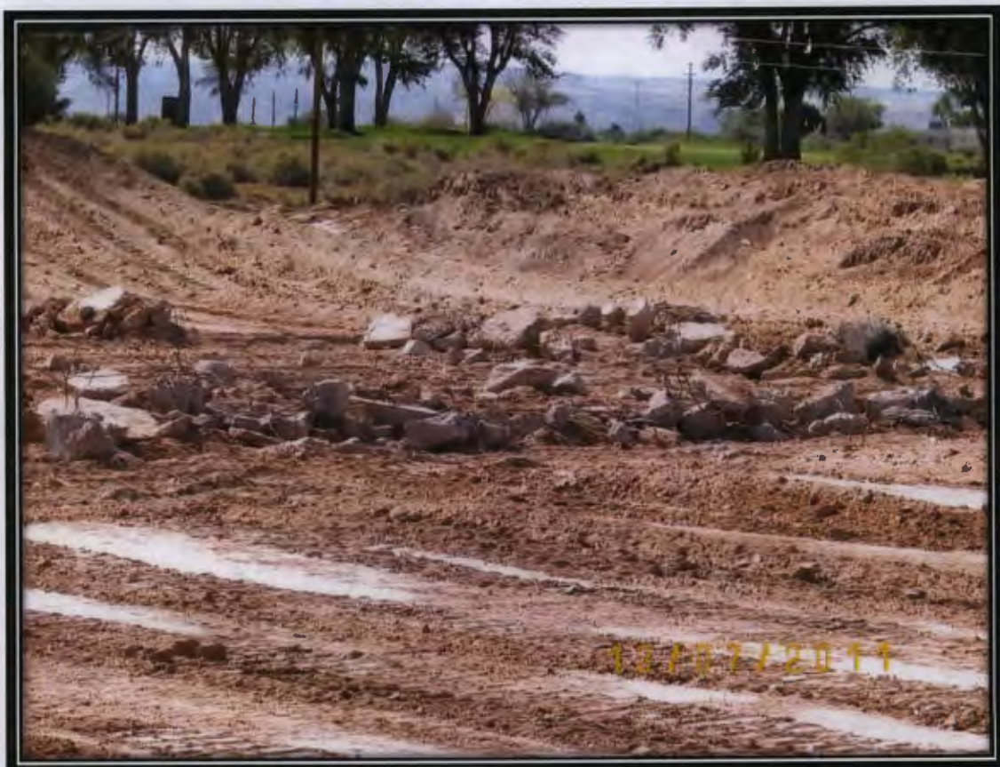
Photo 19 - Placement of Concrete in Former Pit Bottom
