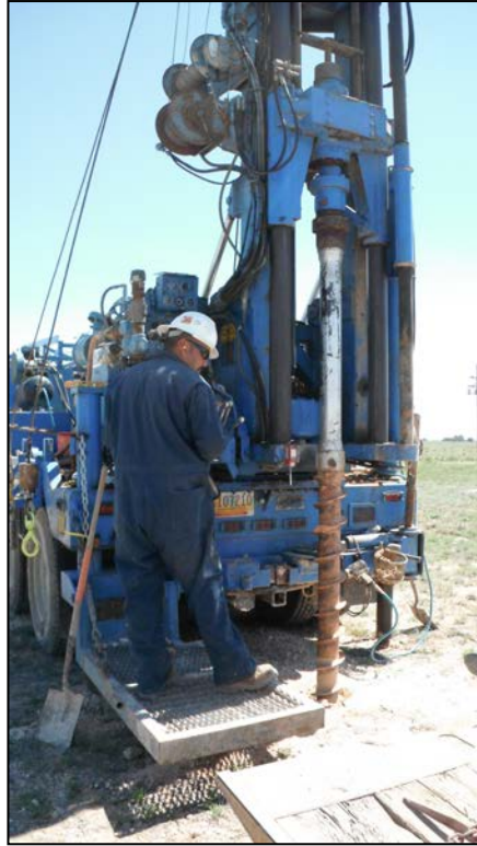
No. 1 – Setting up over soil boring to begin drilling using HSA drilling methods.
