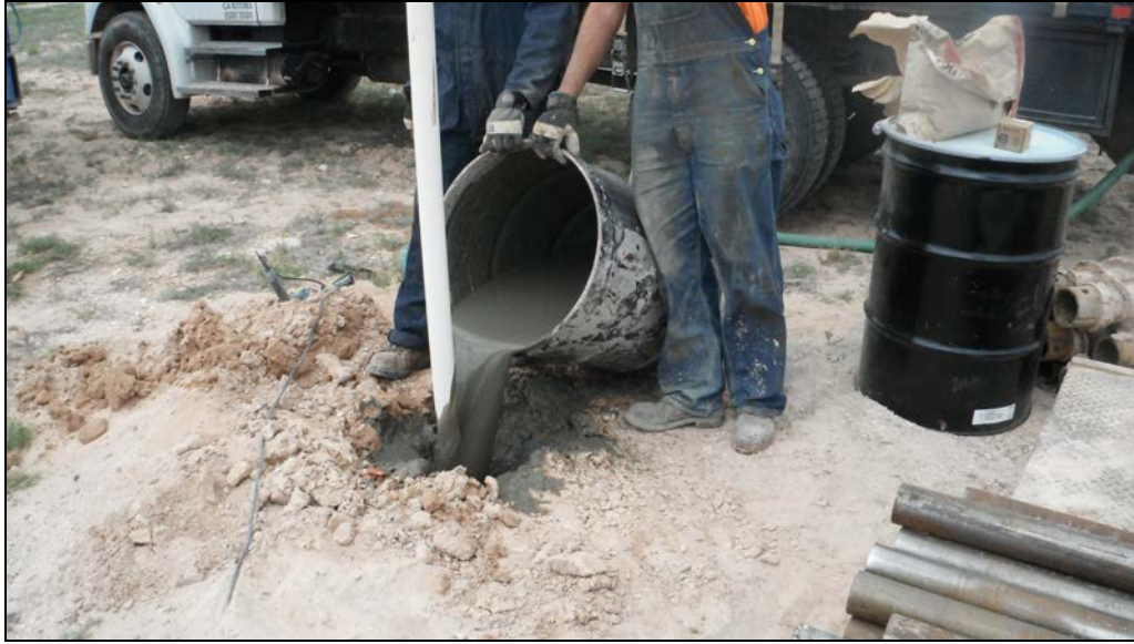
No. 7 – View of cement/bentonite grout being installed at a monitoring well location.
