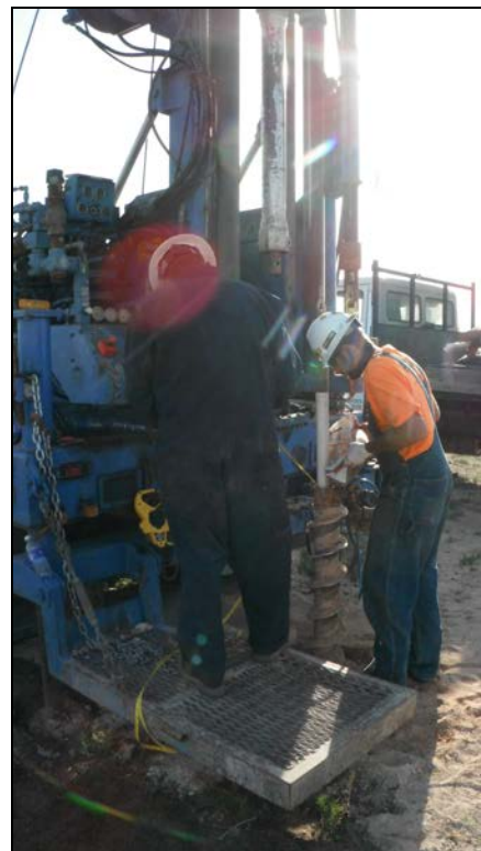
No. 6 – View of filter pack installation at a monitoring location.
