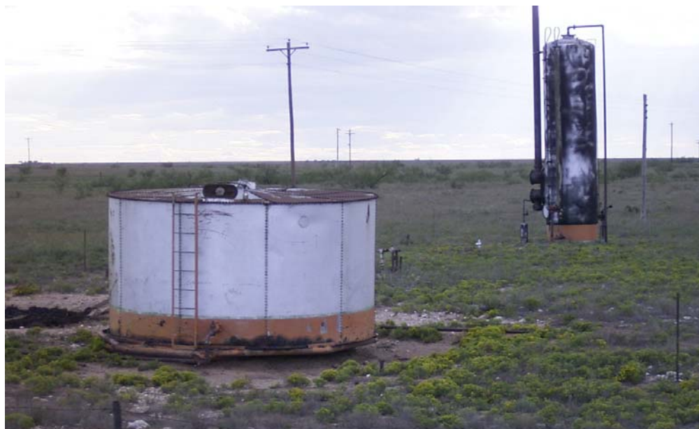
Figure 3. A 210-Barrel Bolted Steel Tank The tank bottom is corroded and the soils below and adjacent to the tank are stained.
