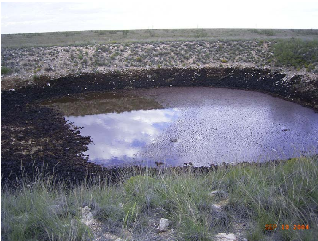
Figure 13. The Reserve Pit, Containing Oil, Water, and Sludge With Contaminated Soils
