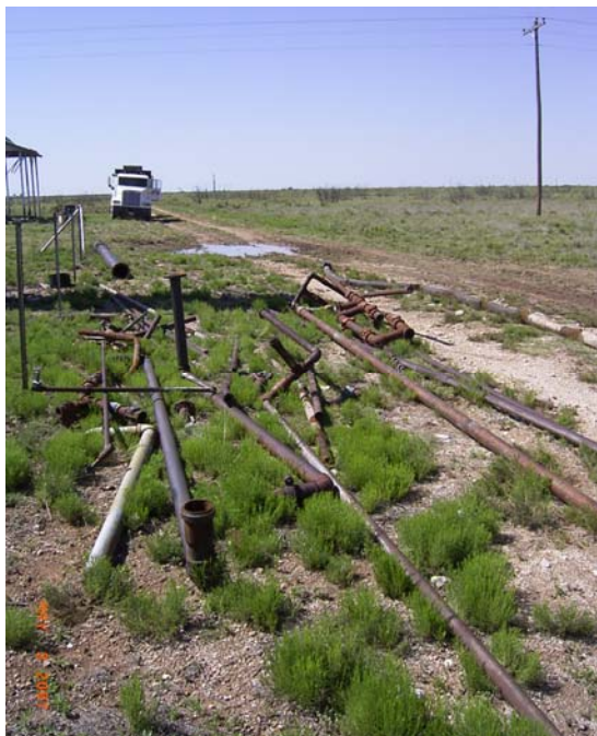
Figure 9 (left): Piping Ready For Removal and Disposal
