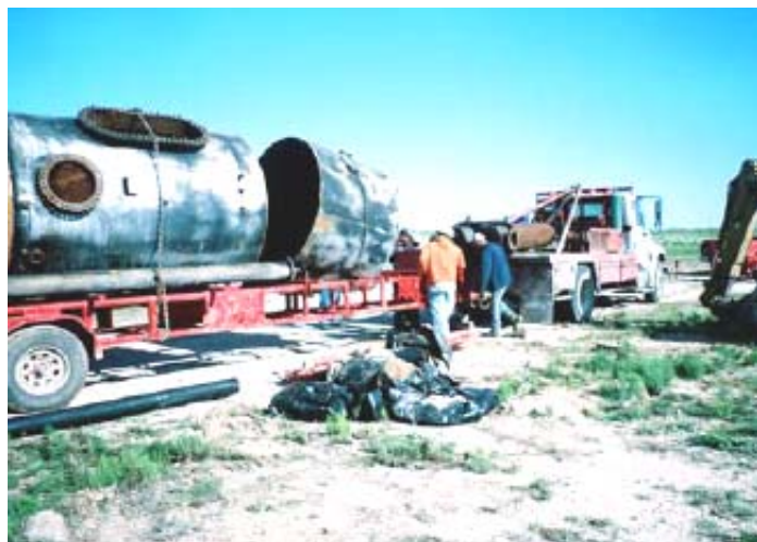
Figure 6. Heater Treater Being Cleaned
