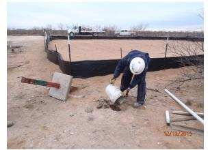
Plugging MW-1 with a 1-3% bentonite-concrete slurry and a 3 ft concrete cap, facing west 12/12/13
