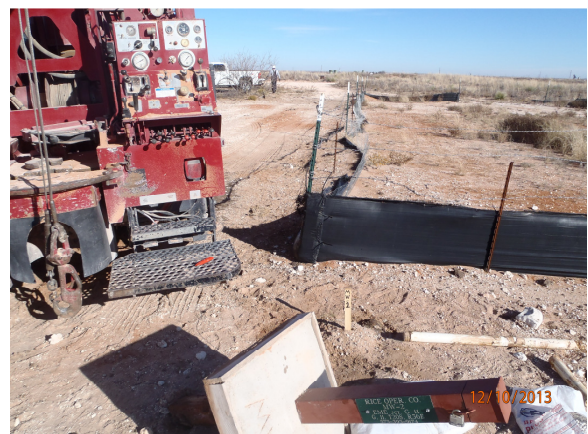
Completed plug and abandon of MW-2, facing east 12/10/13
