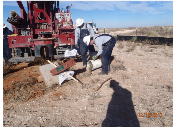
Plugging MW-1 with a 1-3% bentonite-concrete slurry and a 3 ft concrete cap, facing northeast 12/10/13
