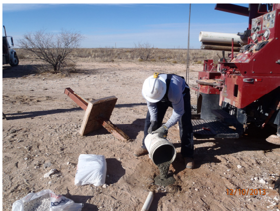
Plugging MW-2 with a 1-3% bentonite-concrete slurry and a 3 ft concrete cap, facing northeast 12/10/13
