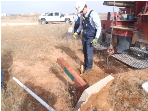
MW-3 plugged and abandoned, facing north 12/10/13
