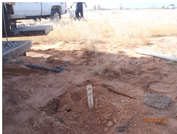
MW-6R plugged and abandoned, facing southwest 12/10/13
