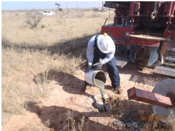
Plugging MW-4 with a 1-3% bentonite-concrete slurry and a 3 ft concrete cap, facing east 12/10/13
