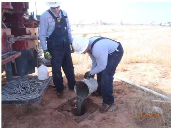
Plugging MW-6R with a 1-3% bentonite-concrete slurry and a 3 ft concrete cap, facing east 12/10/13
