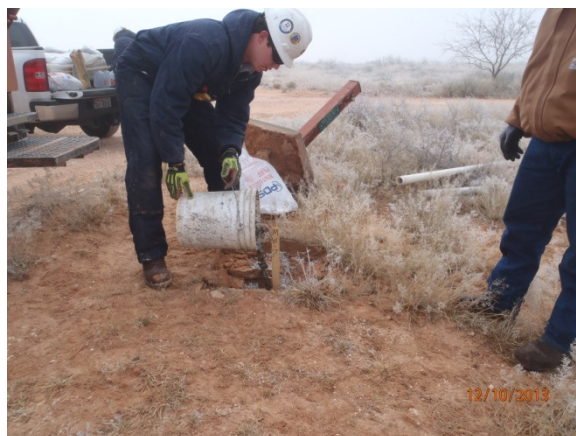
Plugging MW-7 with a 1-3% bentonite-concrete slurry and a 3 ft concrete cap, facing east 12/10/13
