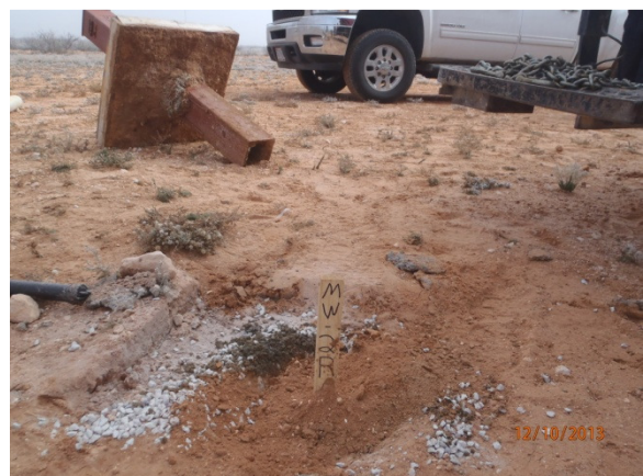
MW-2R plugged and abandoned, facing west 12/10/13
