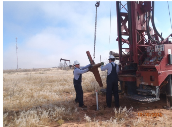
Pulling MW-6R, facing northeast 12/10/13
