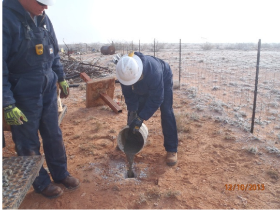
Plugging MW-8 with a 1-3% bentonite-concrete slurry and a 3 ft concrete cap, facing east 12/10/13
