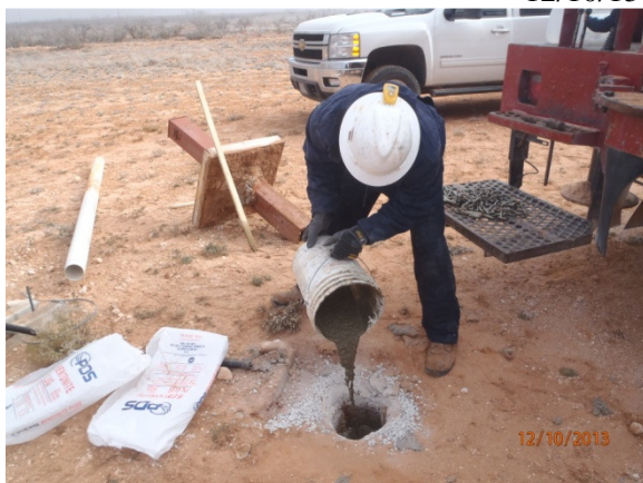
Plugging MW-2R with a 1-3% bentonite-concrete slurry and a 3 ft concrete cap, facing west 12/10/13
