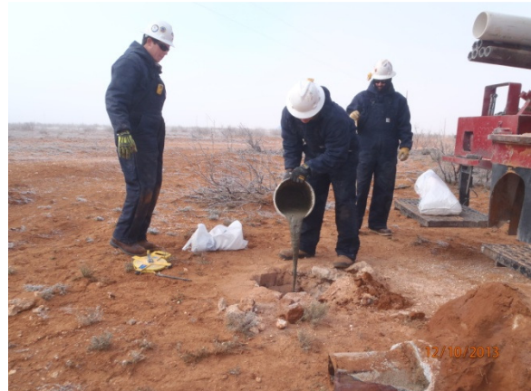
Plugging MW-1 with a 1-3% bentonite-concrete slurry and a 3 ft concrete cap, facing west 12/10/13
