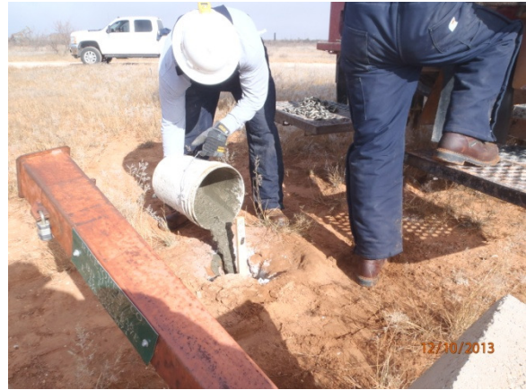
Plugging MW-3 with a 1-3% bentonite-concrete slurry and a 3 ft concrete cap, facing north 12/10/13
