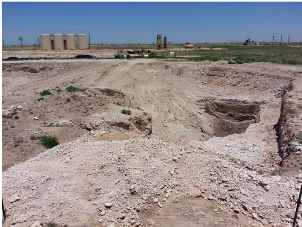
East Side of Excavation Viewing North, July 9, 2013
