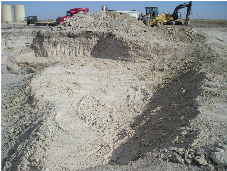
East Side of Excavation Viewing North, October 4, 2012
