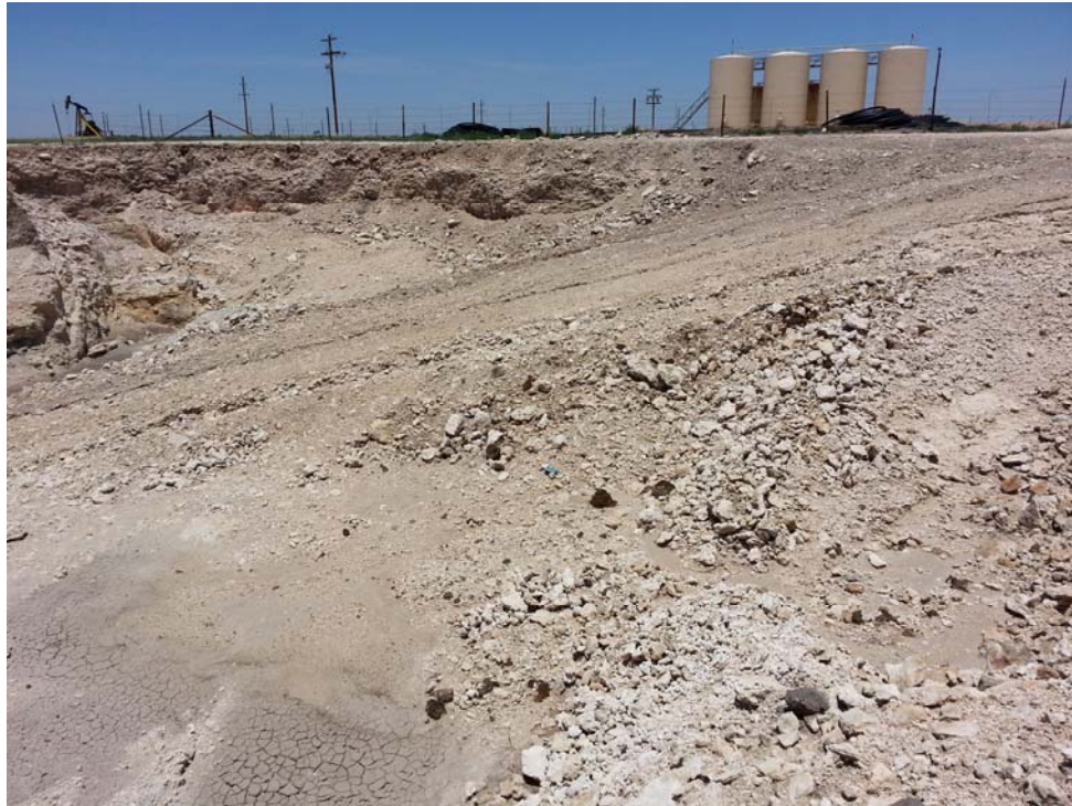
Central Area of Excavation Viewing North, July 9, 2013
