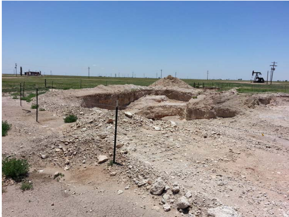
East Side of Excavation Viewing South, July 9, 2013
