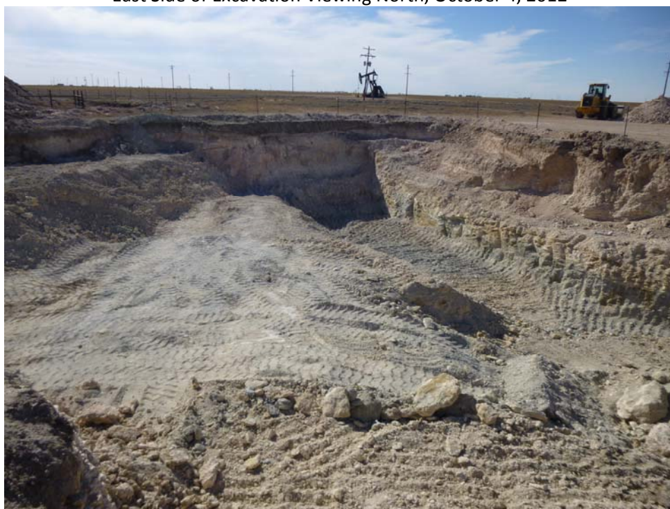
Southwest Corner of Excavation Viewing Southwest, October 4, 2012
