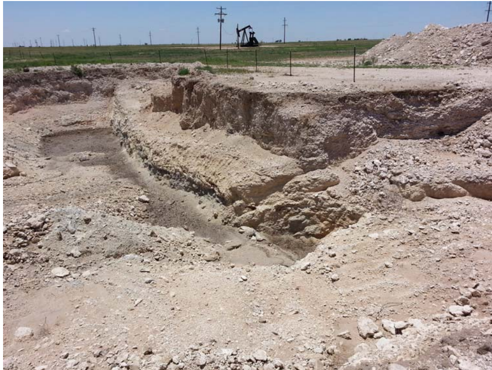
West Side of Excavation Viewing South, July 9, 2013
