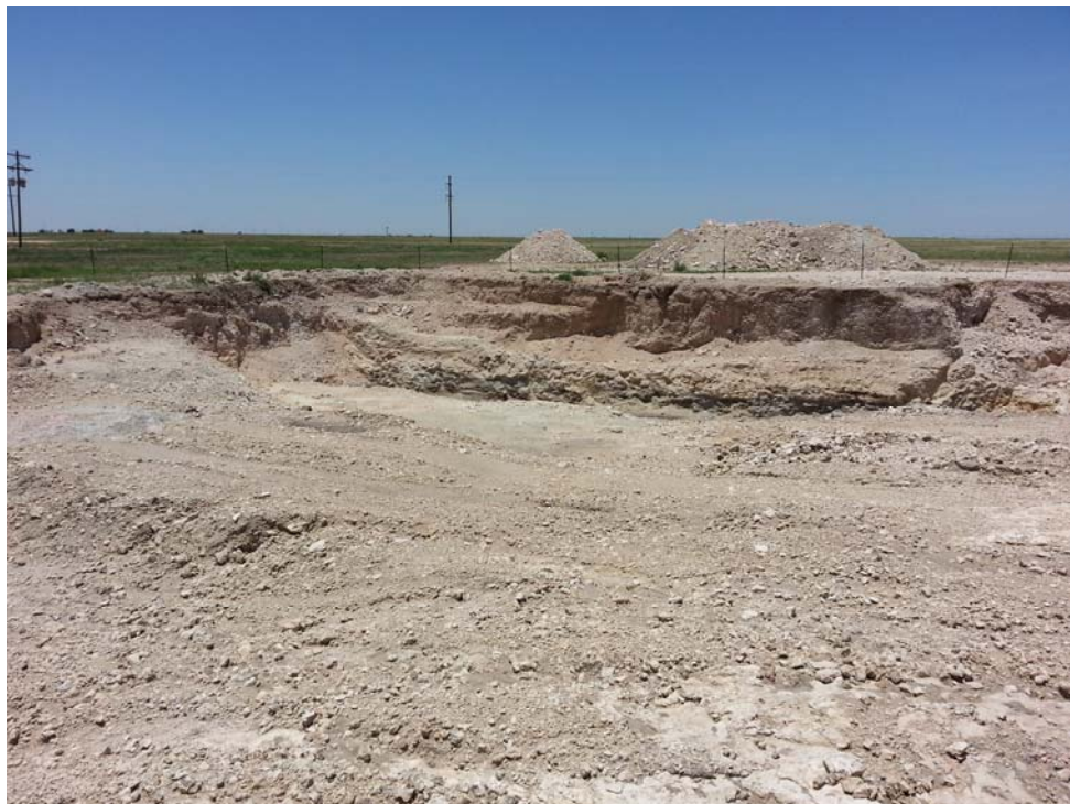
West Side of Excavation Viewing West, July 9, 2013
