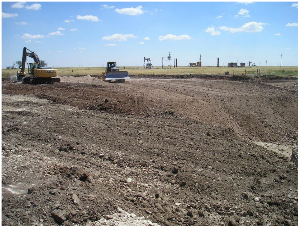
Preparing Excavation for Liner Viewing South, September 4, 2013
