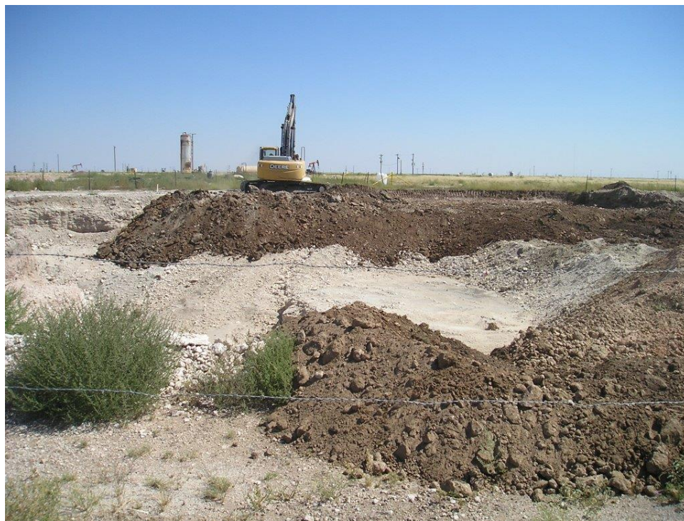
Preparing Excavation for Liner Installation Viewing East, September 4, 2013
