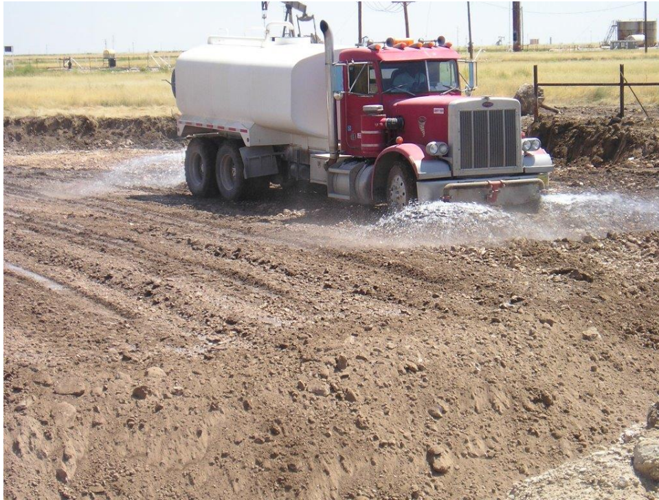
Preparing Excavation for Liner Viewing Southeast, September 4, 2013
