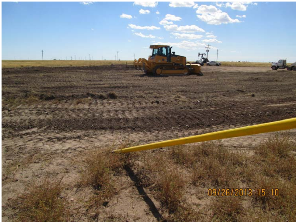
Grading after Liner and Topsoil Viewing Southwest, September 26, 2013
