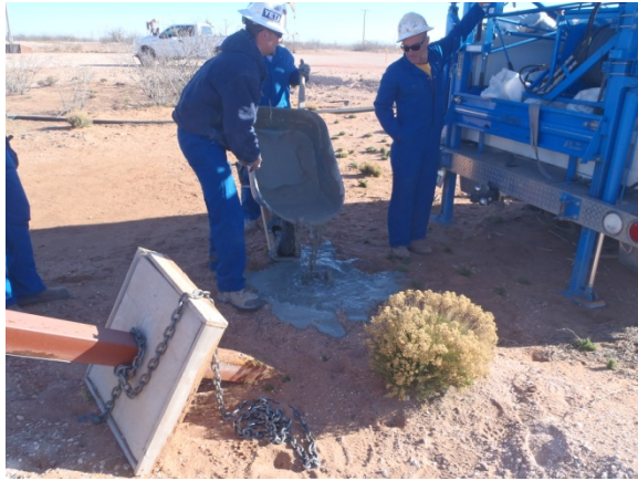
Plugging MW-2 with 1-3% Bentonite/concrete slurry with a 3ft concrete cap, facing northeast 03/05/14
