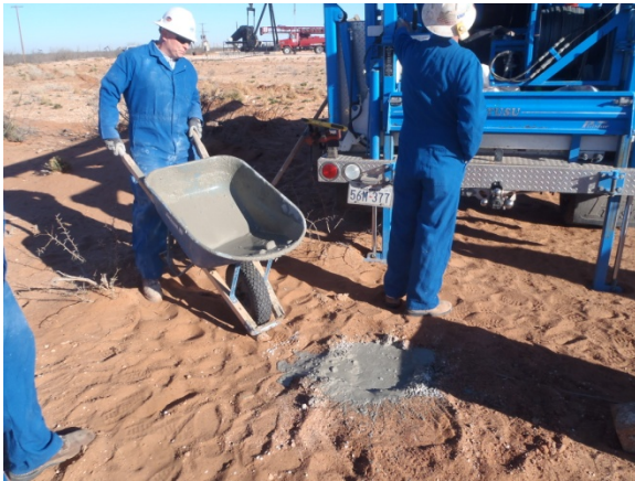
Plugging MW-1 with a 1-3% bentonite/concrete slurry with a 3ft concrete cap, facing northwest 03/05/14
