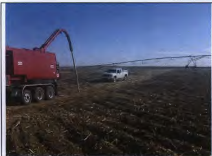
1.) General view of hydro-vac activities to "day light" the pipeline prior to drilling.
