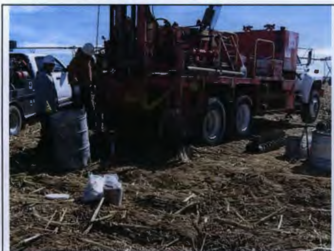
3.) General view of monitoring well installation activities.
