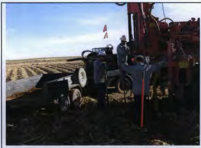
2.) Representative view of soil boring advancement.
