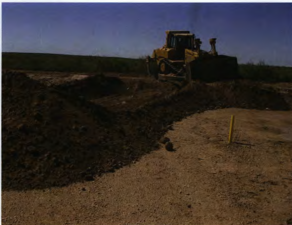
Figure 1: Stockpiling chloride impacted caliche near western 1/3 of location pad.
