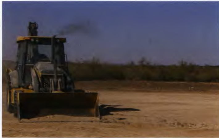
Figure 2: Backfilling a "Y" shaped trench with caliche.
