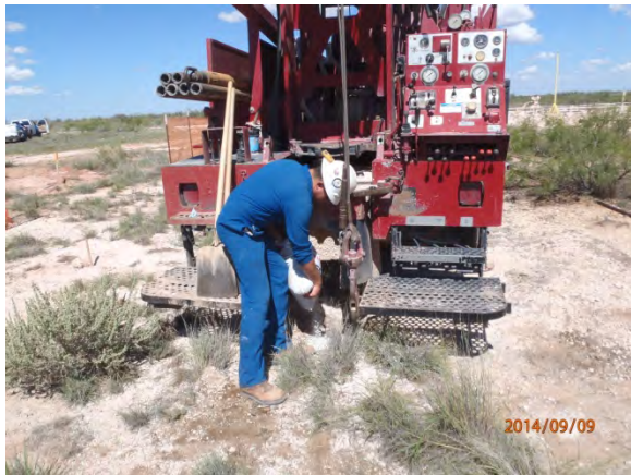
Plugging SB-7 in total with bentonite 09-9-14
