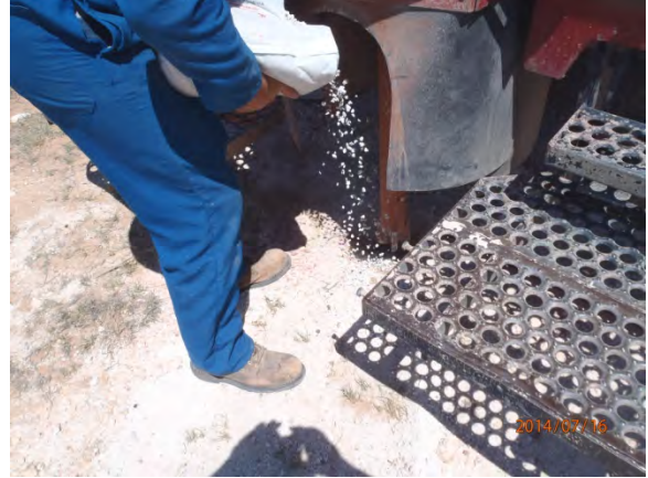
Plugging SB-6 in total with bentonite 07-16-14
