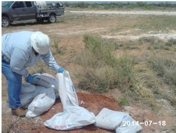
Plugging SB-2 in total with bentonite 07-18-14
