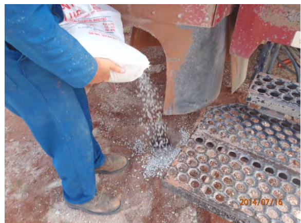
Plugging SB-3 in total with bentonite 07-16-14
