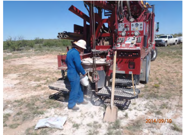
Plugging SB-10 in total with bentonite 09-10-14
