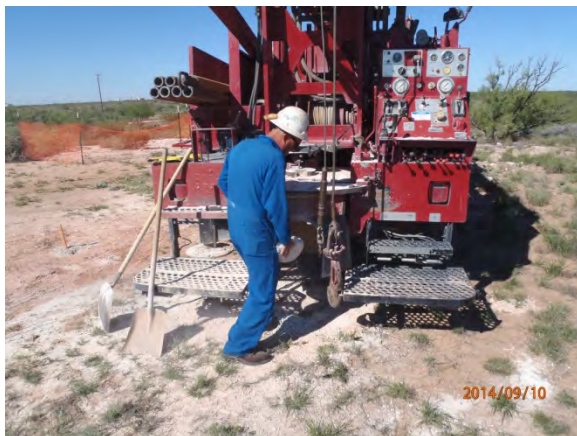
Plugging SB-9 in total with bentonite 09-10-14
