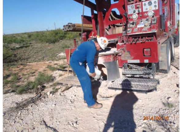
Plugging SB-8 in total with bentonite 09-09-14
