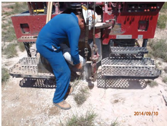
Plugging SB-11 in total with bentonite 09-10-14
