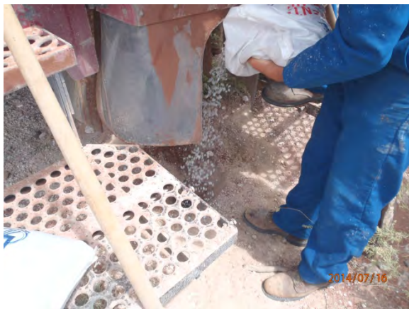
Plugging SB-4 in total with bentonite
