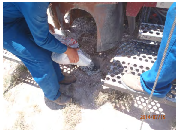
Plugging SB-5 in total with bentonite
