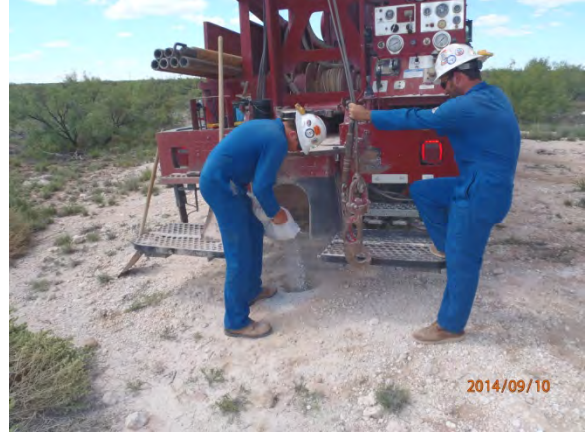
Plugging SB-12 in total with bentonite 09-10-14
