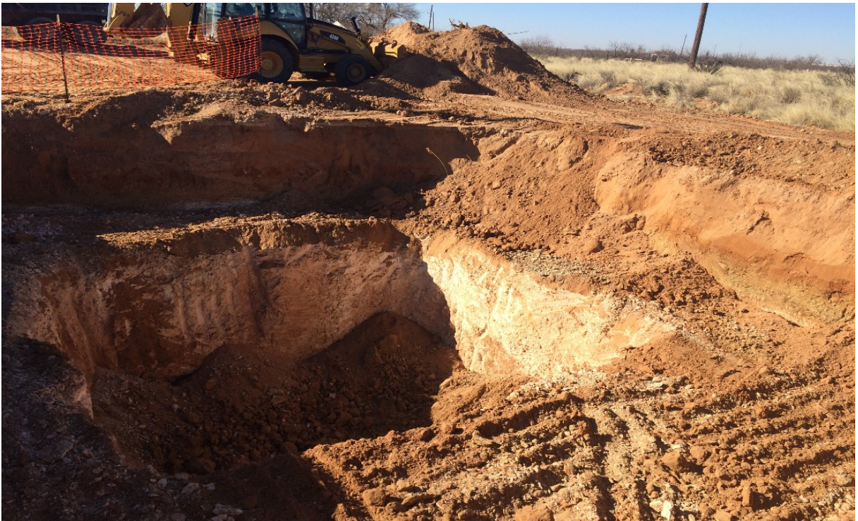
View Southwest - Benched Area and Excavated Depth
