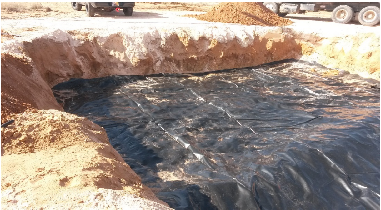
View Southwest – Liner Installed
