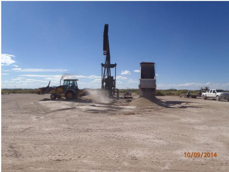
Importing caliche and backfilling scrape, facing west
