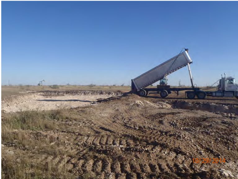
Importing top soil to pad for liner, facing north 10/29/14
