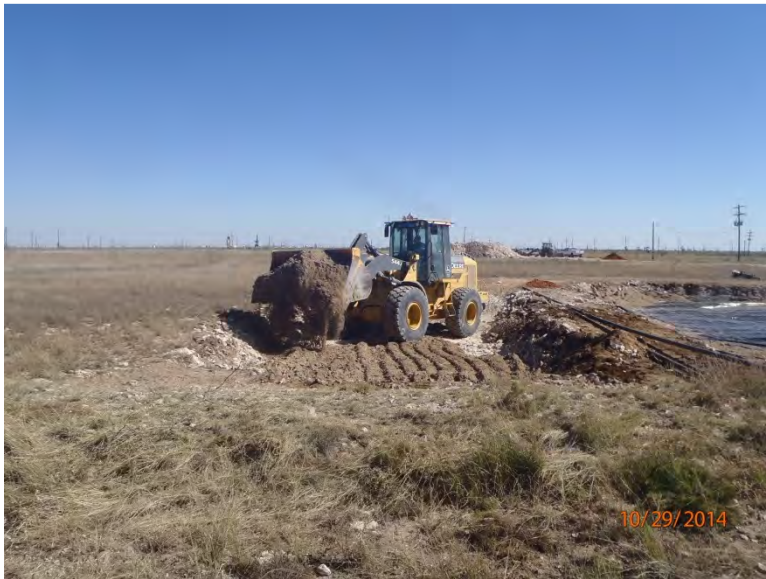
Padding north excavation (2) for liner installation, facing east 10/29/14
