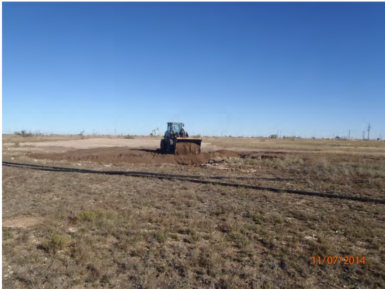
Backfilling south excavation, facing northeast
