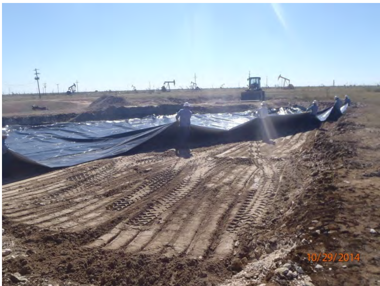
North excavation padded with imported soil and installing liner, facing southeast 10/29/14
