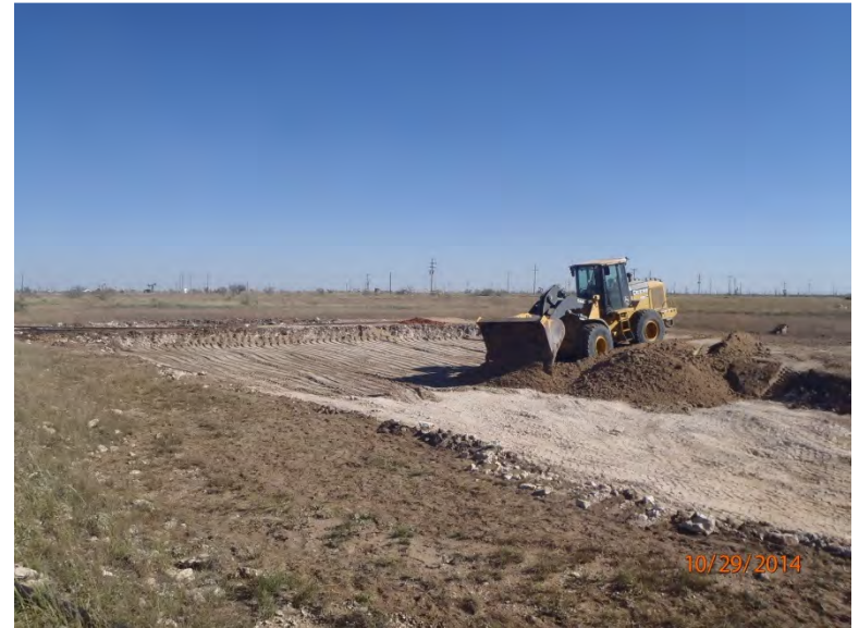
Padding north excavation for liner installation, facing northeast 10/29/14
