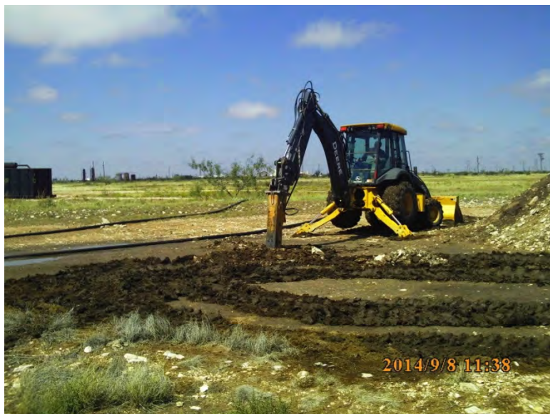
Installing verticals, facing northwest
