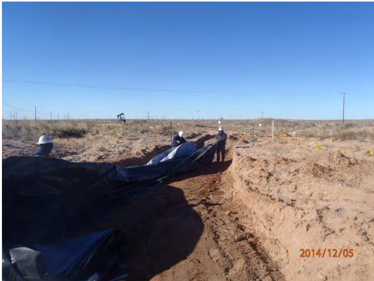
Installing liner, facing southwest
