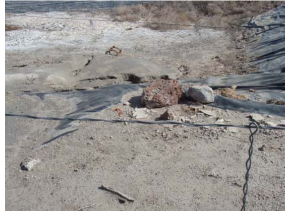
LDG 47-7 Drill Pit with Stormwater Sediments & Rocks Inside Pit
