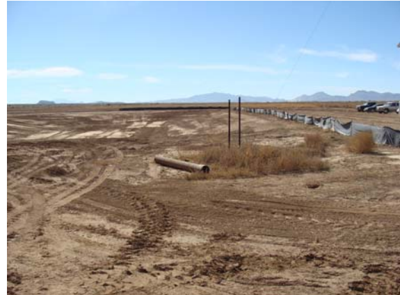
Recently Constructed Run-Off Pond at SW Area of Property with Silt Fence Along W & S Perimeter of Pond Controlling Stormwater Drainage Across Facility from E to W
