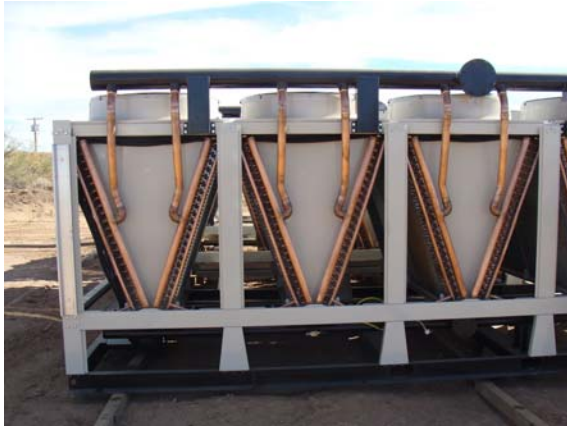
Air-based Cooling Tower Unit
