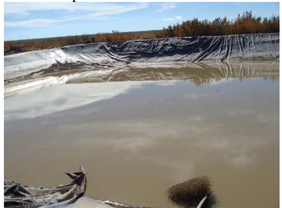
Looking W at Central Evaporation Pond Stormwater Damage Along Berms Evident with Torn Liner
