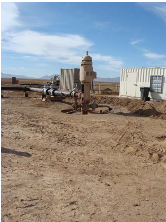
Production Well LDG 45-7 Well Head with 400 HP Pump
