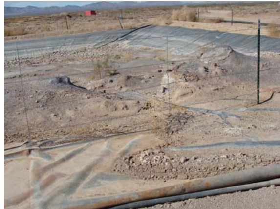
LDG 63-7 Drill Pit and Stormwater Sediments Deposited Inside Pit
