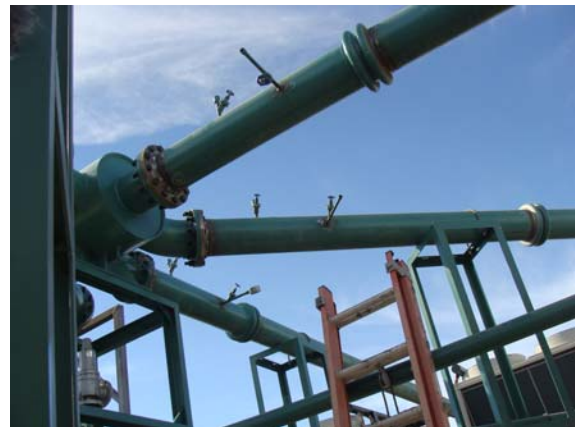
Power Block 1 of 4 Soap & Water Leak Testing Process Lines
