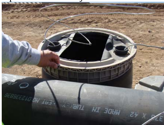
LDG 45-7 ASTM Sample Cooler Near Pipeline Sample Port
