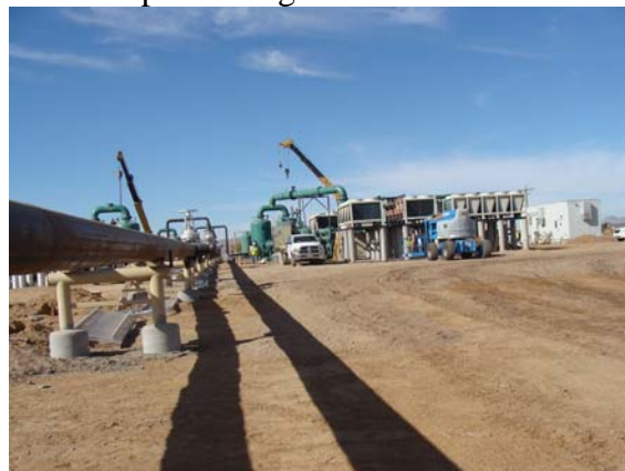
Above ground pipelines: Inlet & Return
