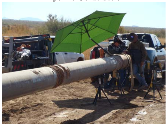
Welder at Pipe Joint
