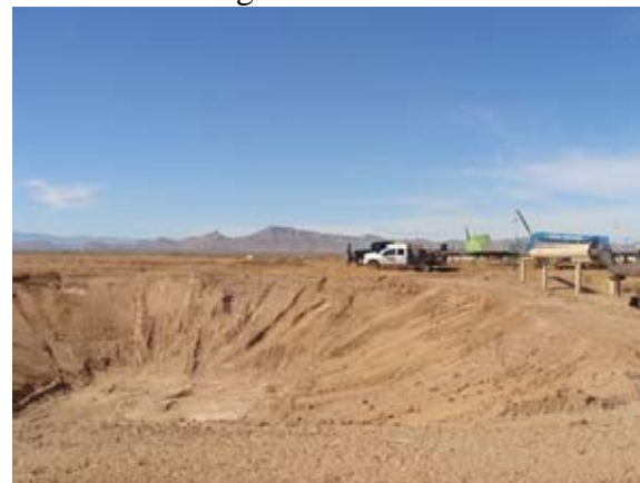
New Blowdown Pit Depression Located Near Each Production/Injection Well for Workovers, etc
