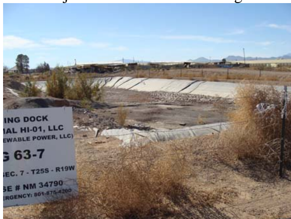
LDG 63-7 Drill Pit with Stormwater Sediments running into pit from berm with vegetation growth inside pit
