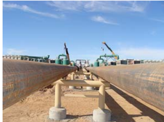
Looking W at Pipelines: Power Plant Input & Return Pipeline to Injection Wells
