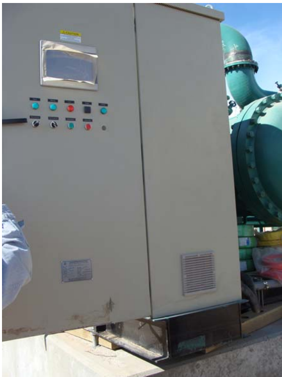
Expander Unit Electric Control Circuit Panel Exterior
