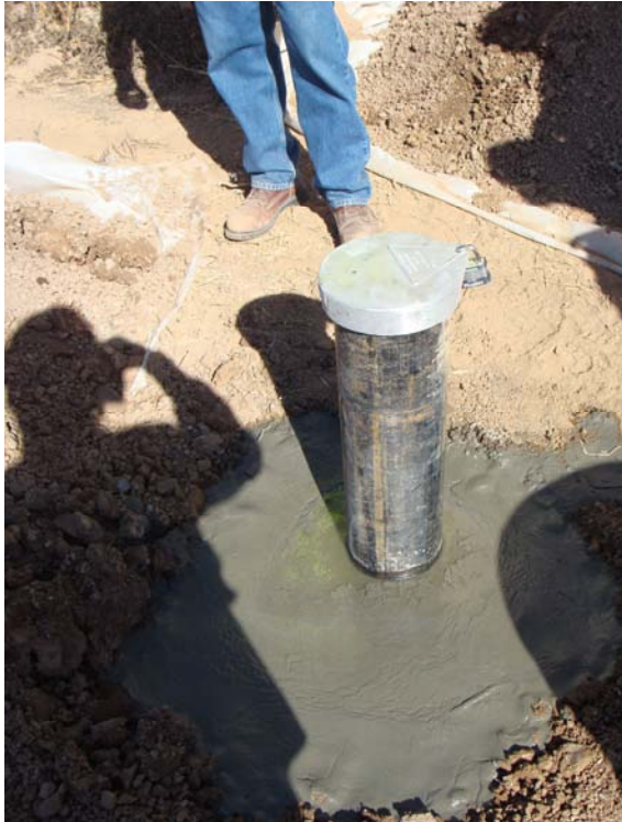
INW-1 (Intermediate Nested Well ~ 600 Ft. Deep) Located Between LDG 45-7 & LDG 55-7
