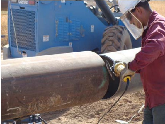
Preparing pipeline joints for welded connection
