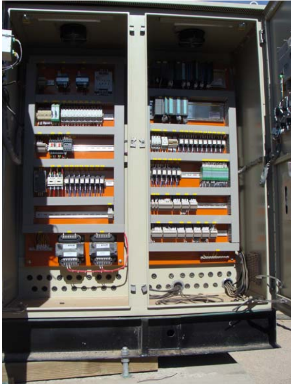
Expander Unit Interior Electric Control Circuit Panel 1250 V
