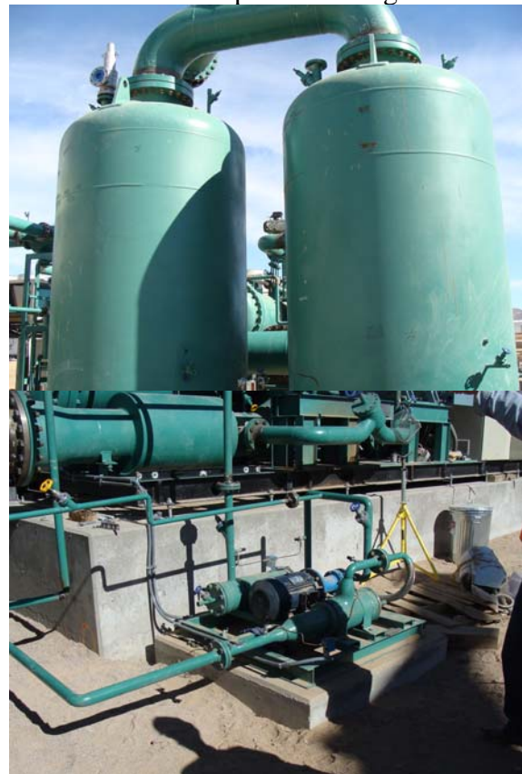
Block 1 of 4 Oil Separator Refrigerant Side
