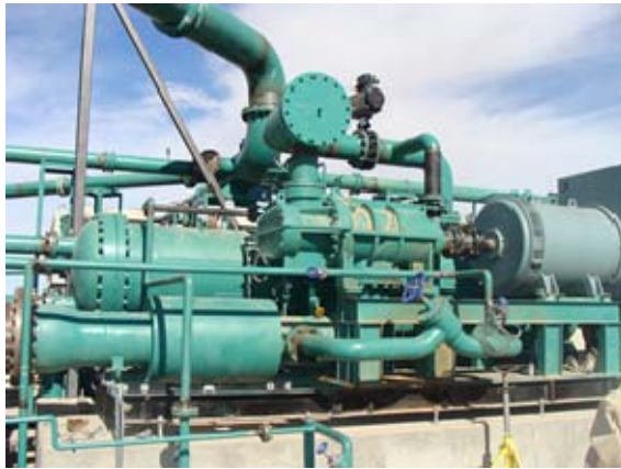
Block 1 of 4 Kaishan Turbine Screw Expander Unit (1.2 MW)
