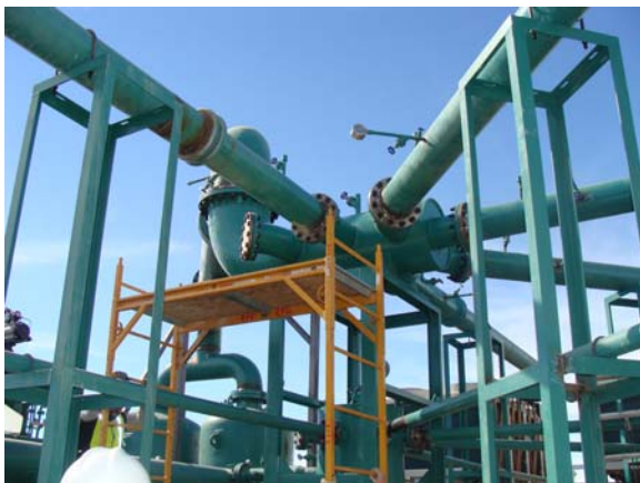
Power Block 1 of 4 Radial Process Lines Extending from Cooling Tower Units to Collector Unit Below
