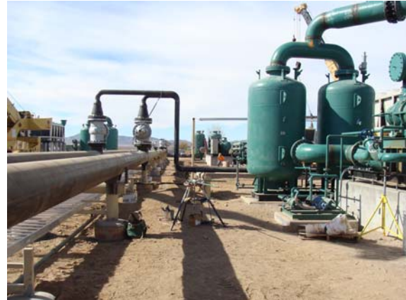
Looking W at Produced Fluid Pipelines: Intake Pipeline from Production Well LDG 45-7 Tie-In to Block 1 and all 4 Power Plant Blocks under Construction with Return Pipeline (Eastward) back to Injection Wells
