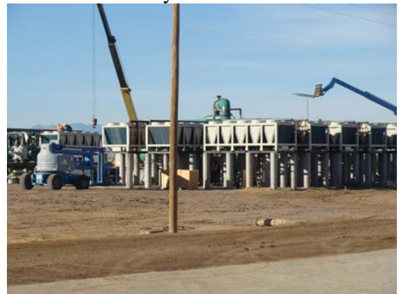
Looking SW at Block 1 of 4 power plant with air-based cooling tower system placed on top of 7 foot piers
