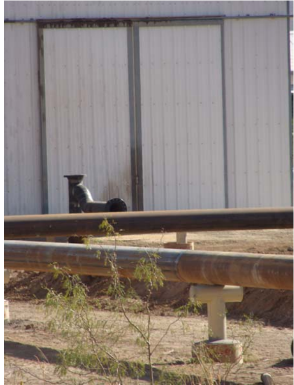
Elevated pipeline (uninsulated)
