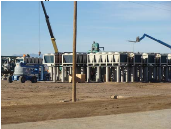
Looking SW at power plant and air-based cooling towers in first of four constructed blocks (Ea. ~ 1.2 MW)
