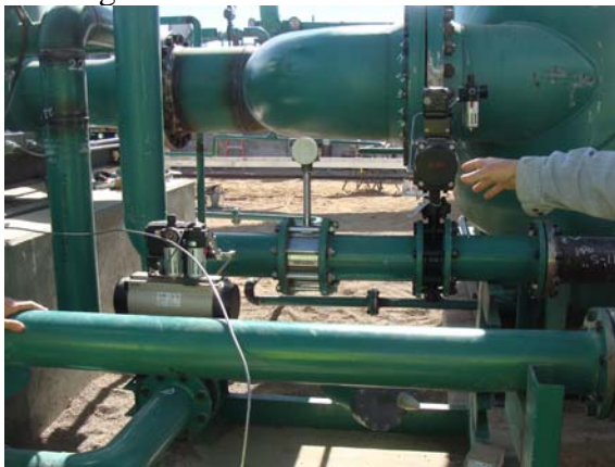
Block 1 of 4 Oil Separator Refrigerant Level Indicator
