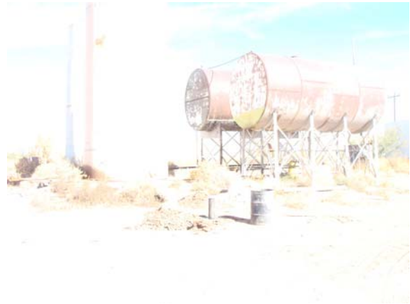
Above Ground Fuel Storage Saddle Tanks without Secondary Containment
