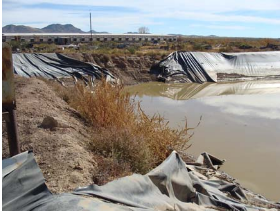
Looking S-SE at Central Evaporation Pond Liner Tears along E and SE berm areas
