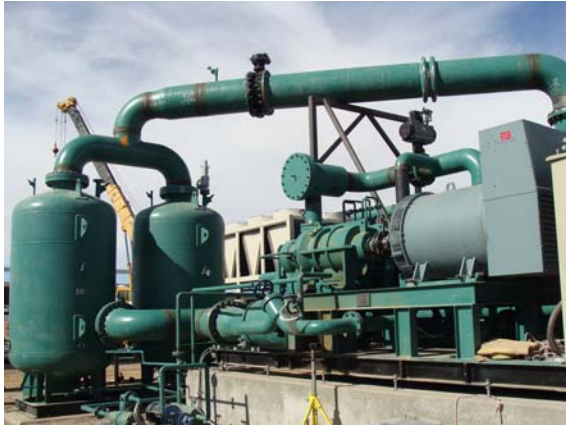
Block 1 of 4 Oil Separator Refrigerant Side of Expander Unit
