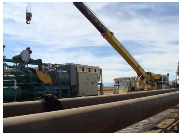
Looking SW Pipelines (Intake & Return) from Production Well LDG 45-7 Feeding into all 4 Power Plant Blocks with Block 2 of 4 Under Construction
