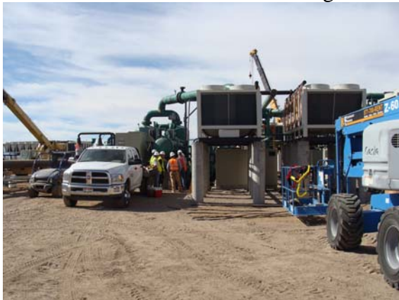
Cooling Tower Units at Block 2 of 4 Under Construction
