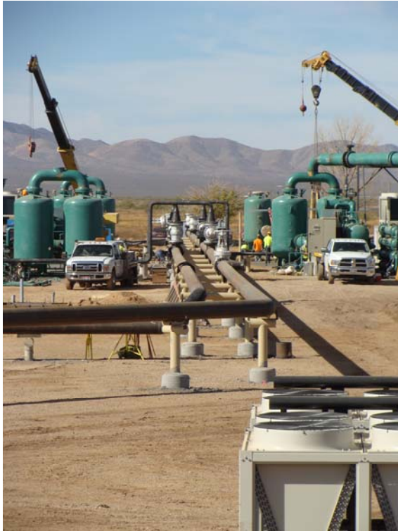
Looking West at oil separators (1 unit per Block) for refrigerant side of each Power Block
