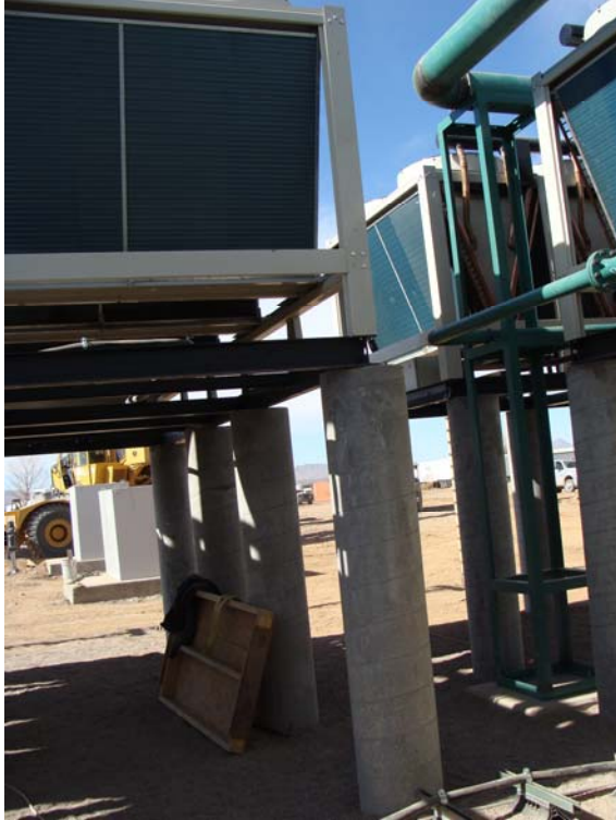
Cooling Tower Units Sit On 7 Ft. Tall Piers
