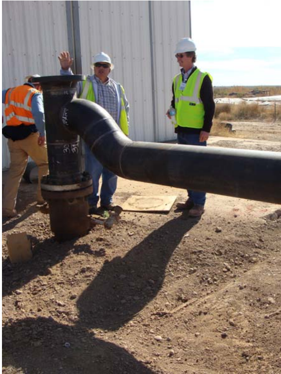
Main Injection Well LDG 55-7 open to environment (uninsulated)
