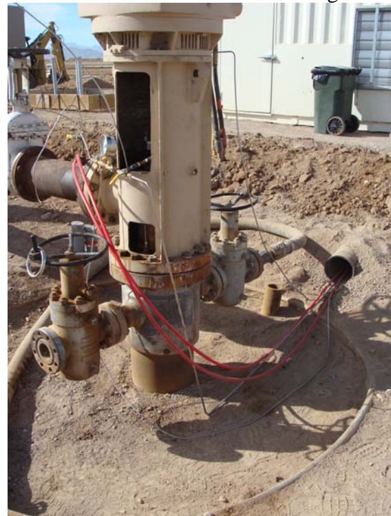
LDG 45-7 Top Mounted Water or Oil-Lubricated? Line Shaft Pump (400 HP)
